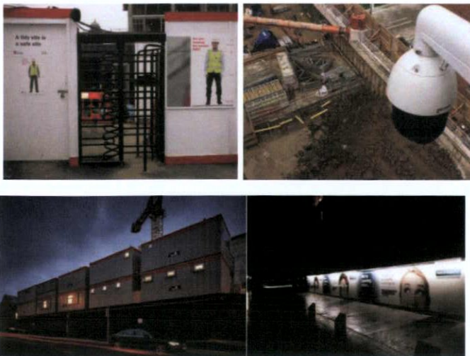
Figure 9 _Typical Site Security Measures
