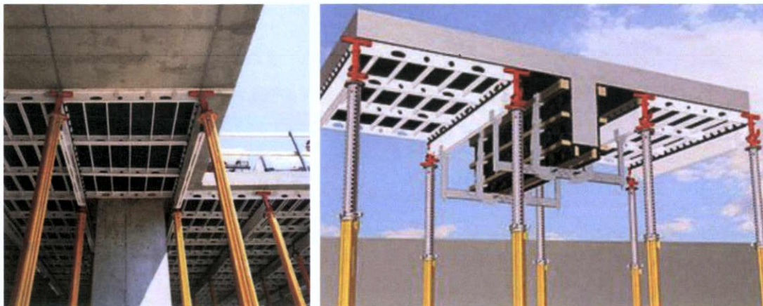
Figure 14 - Typical RC Formwork (Skydeck)
