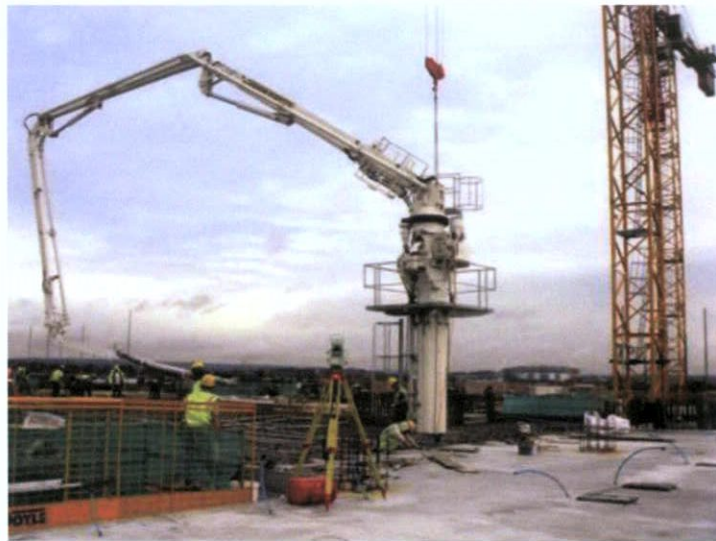
Figure 15 - Typical Concrete Placement
