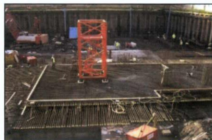
Figure 7 Typical Tower Crane Anchors
