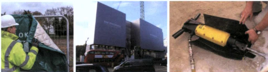
Figure 39 – Typical Noise Mitigation Measures
