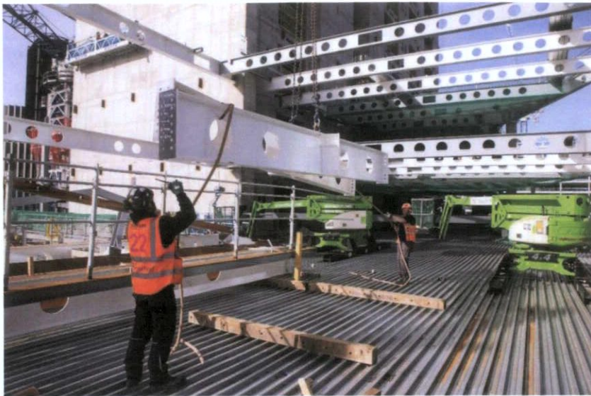
Figure 16 – Typical Steel Frame Erection
