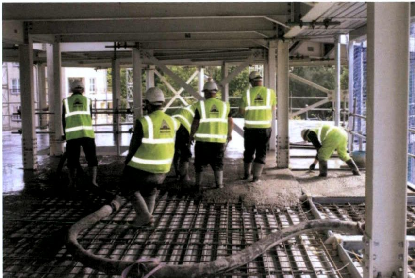
Figure 17 – Typical Concrete Pour on Metal Decking
