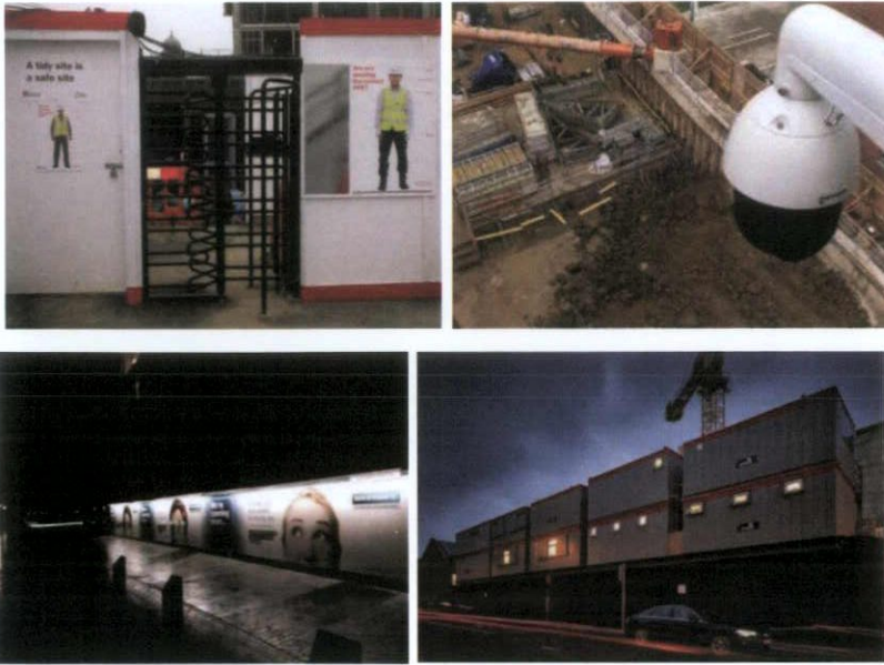
Figure 9 – Typical Site Security Measures
