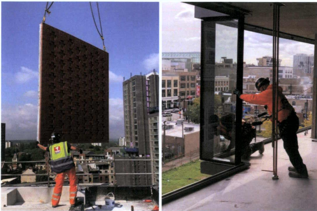
Figure 21 – Typical Precast Concrete Panel & Curtain Wall Panel Installation
