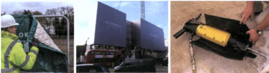
Figure 25 – Typical Noise Mitigation Measures
