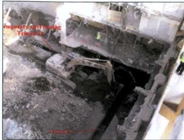
Figure 23 Overview of steel footing trench
