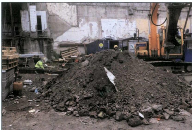
Figure 42 The infill from Trench 4
