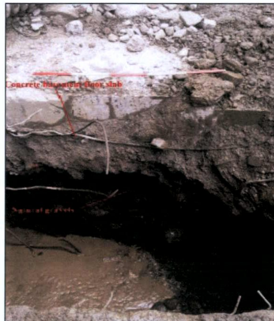
Figure 25 Trench B, concrete and natural gravels
