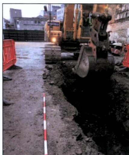
Figure 45 Trench 1, from the east
