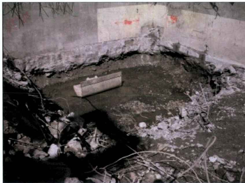
Figure 27 Trench 4, temporary crane base
