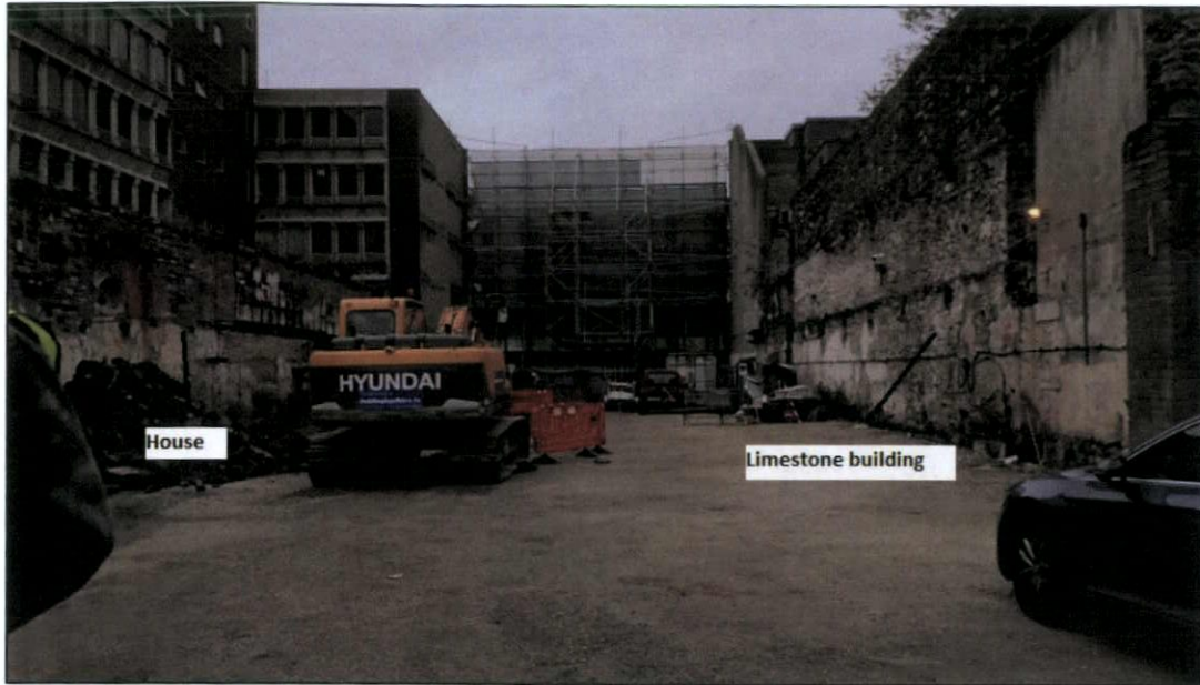
Figure 68 Site from the west
