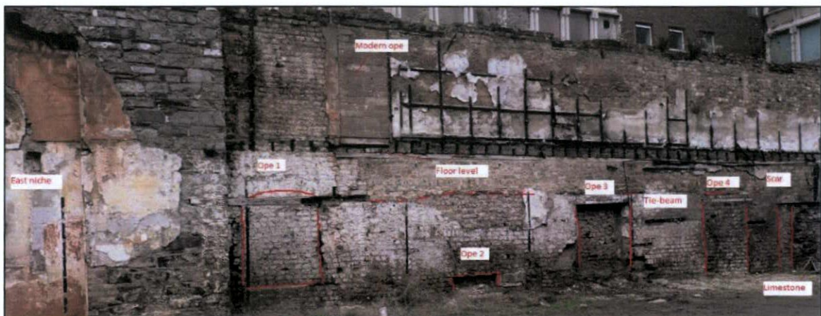
Figure 83 Building 3, from the west
