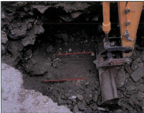
Figure 60 The structure from the north
