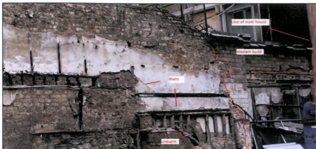
Figure 88 The stairs at the eastern end
