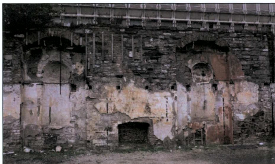
Figure 74 Building 2, from the south
