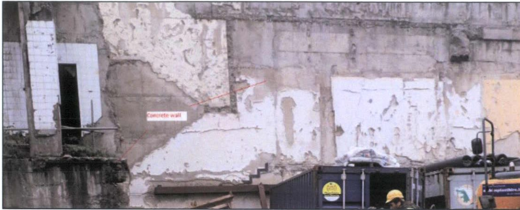
Figure 63 The north wall
