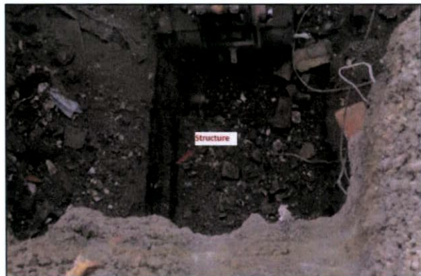
Figure 58 Foundation from the east
