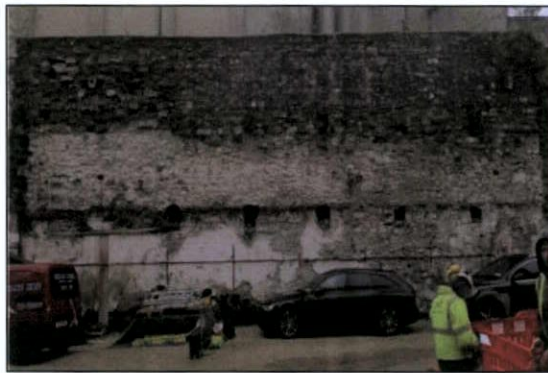
Figure 93 Building 4, from the north
