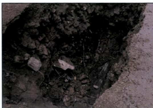
Figure 57 The floor abutting the wall foundation
