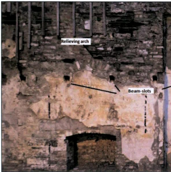
Figure 78 The relieving arch and beam-slots
