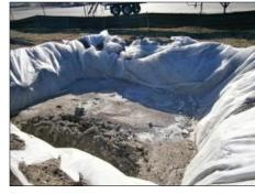
Plate 4-4 Concrete washout area
