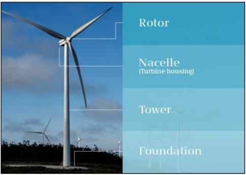
Plate 4-1 Wind turbine components
