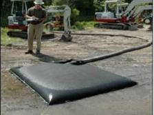
Plate 4-6 Silt Bag with water being pumped through
