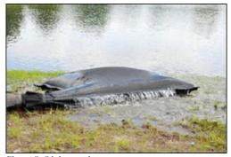
Plate 4-7 Silt bag under inspection
