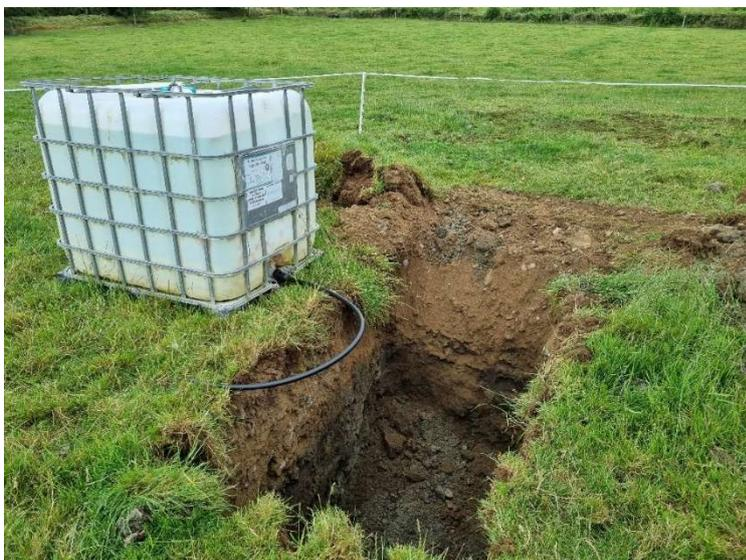
**Plate 6.7 Trial Pit in eastern area of the site – arisings from pit shown**
