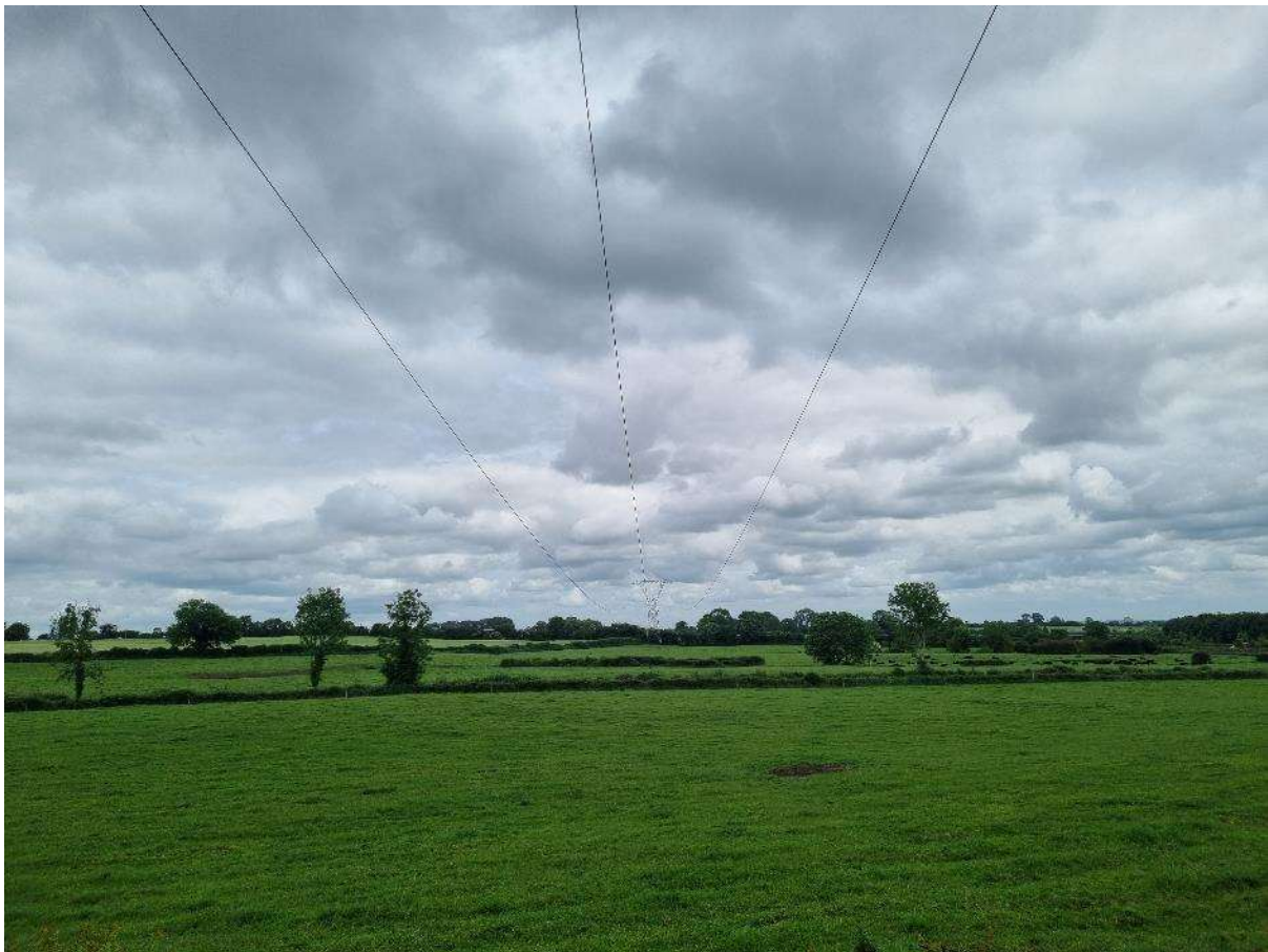
Plate 3.1 Existing 220kV OHL – view east across the site
