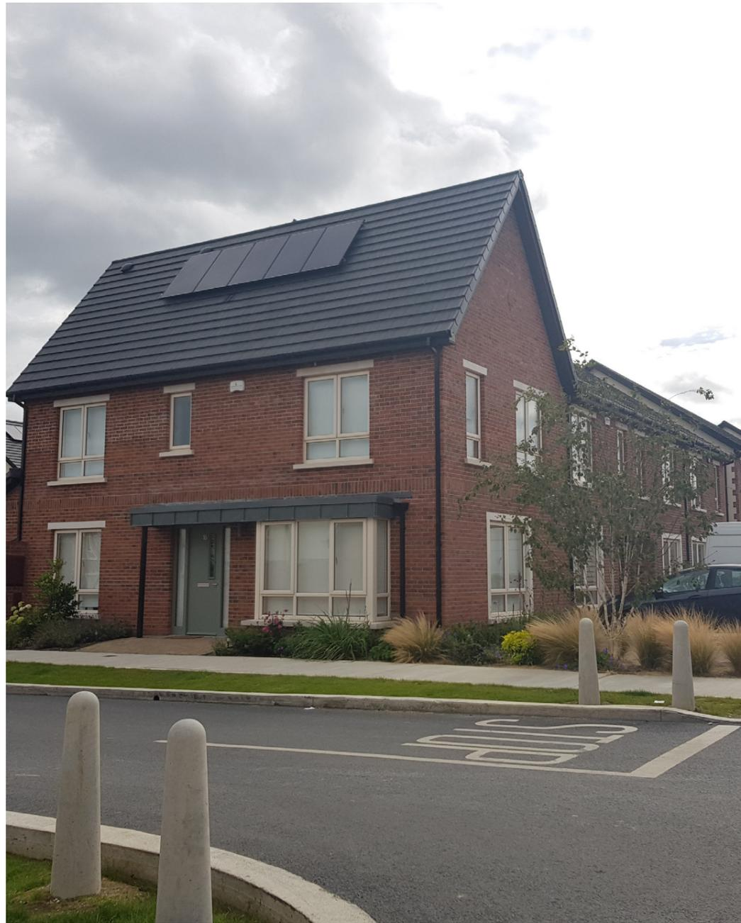
▲ Dual frontage house type used to turn the corner of a street with further animation of bay window & Canopy over front door
