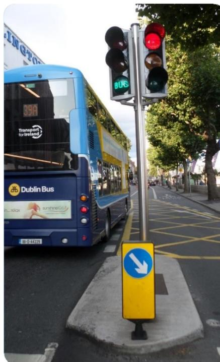
Figure 2: Signal Controlled Bus Priority
