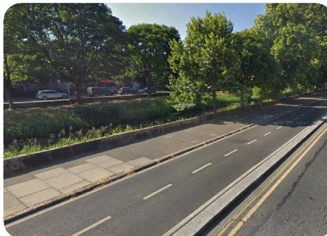
Figure 8: Preferred CBC Cycle facility segregation (example shows a two-way cycle track)
