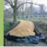
CellWeb™ comprises an expandable cellular mattress that is then filled with a clean stone sub-base and above a Treetex T300 Geotextile.
