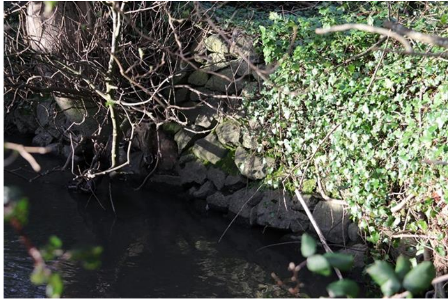
Photo 4: Stone lining on embankment
