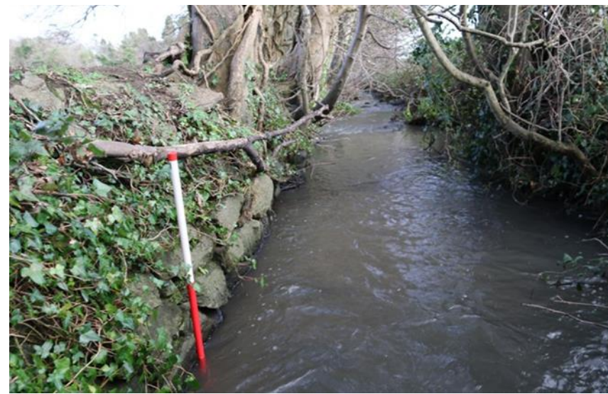
Photo 2: River channel with stone lining
