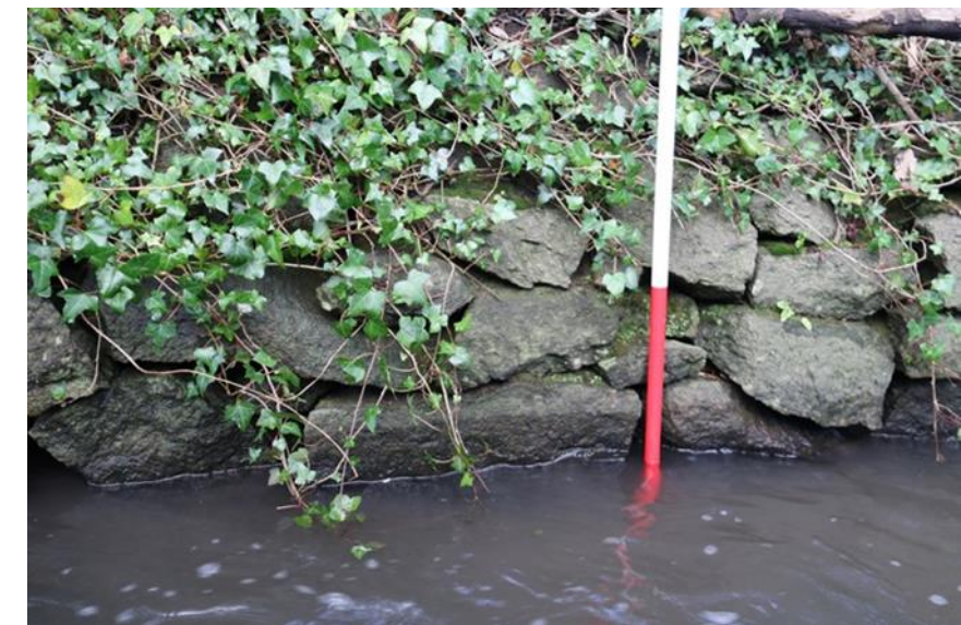
Photo 3: Detail of stone lining
