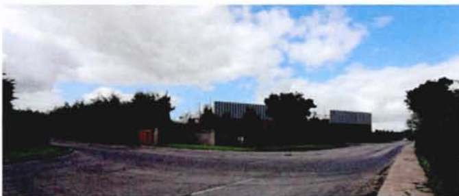
Ground level view from the south-east - 22 September 2020
