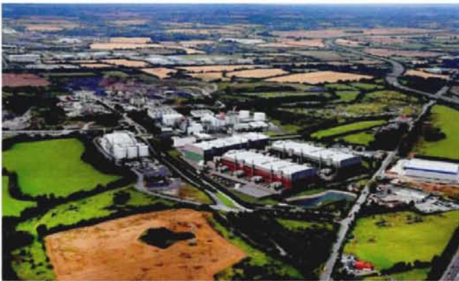
Aerial view from the south - 22 September 2020
