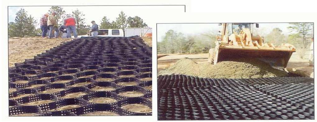
**Pictures show the Cell Web being installed on the ground.**
