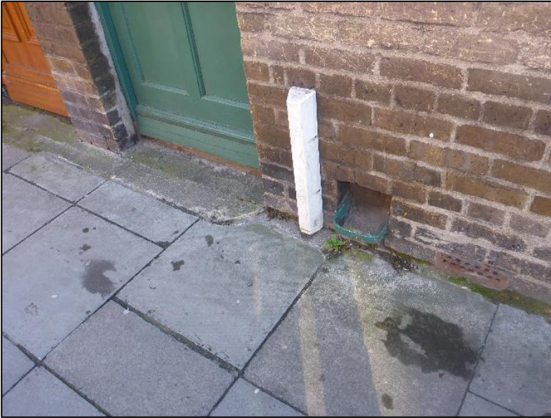
Image 15.20: Boot Scrapes on Blackhall Place
