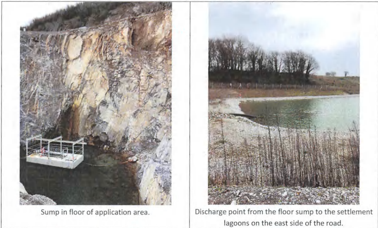
Plate 7.4: Existing discharge mechanism at the site.
