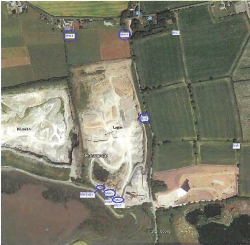
Plate 7.7 Water level monitoring borehole network BHs with blue circle are those which extend deeper than -50mOD
