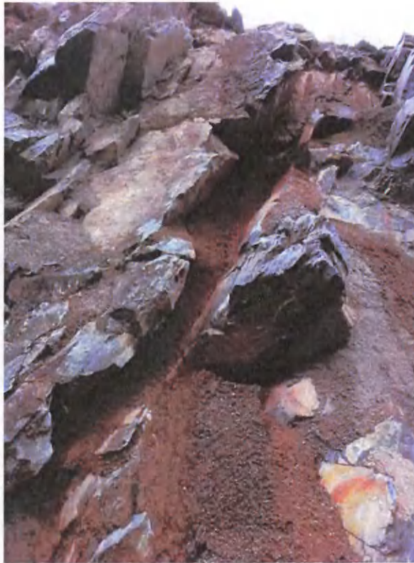
Figure 5 View of central part of western face showing clay infilled joint
