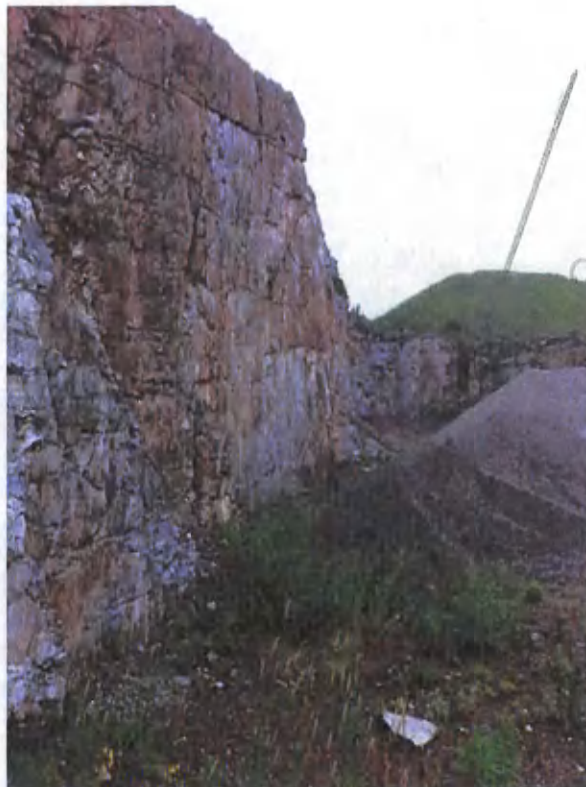
Figure 4 View of central part of western face
