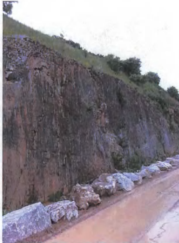
Figure 3 View of southern part of western face
