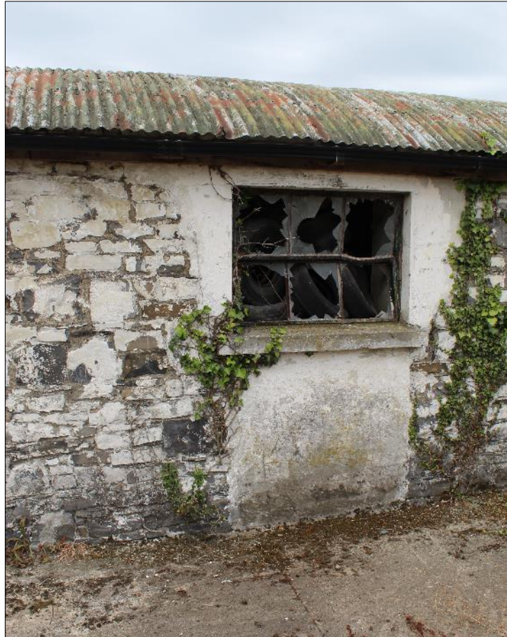
Plate 13.2.11: Detail of altered window opening with concrete sill and infill in rubble calp limestone masonry wall of lower farm building.
