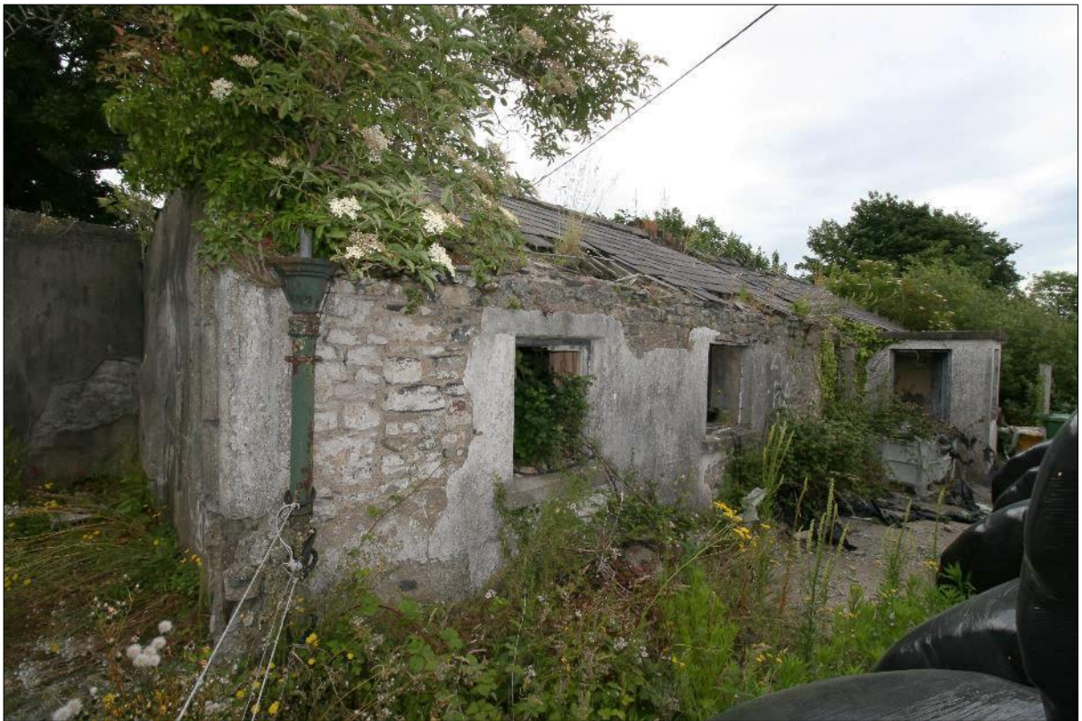
Plate 13.2.6: Front south-west elevation of ruined former dwelling, the windowless rear wall of which forms roadside boundary. Porch is twentieth-century addition and window openings are all enlarged insertions with concrete sills.
