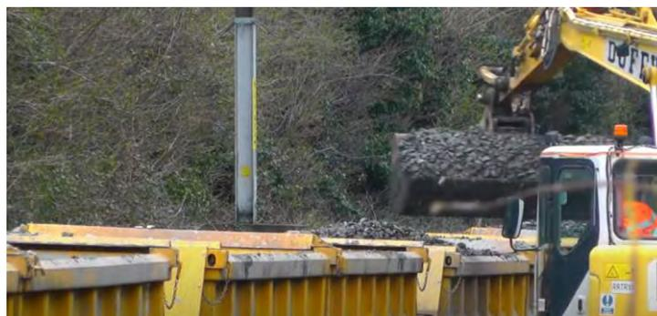
**Figure 5-15 Ballast removal**
