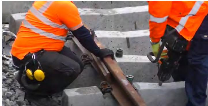
**Figure 5-20 Provisional track panel joint**
