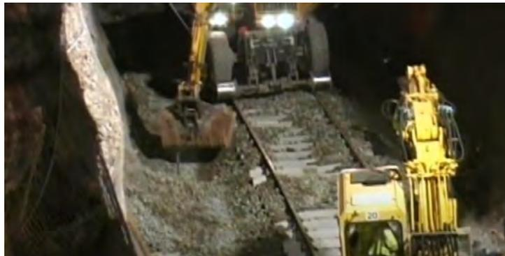
**Figure 5-21 Ballast laying – second layer**
