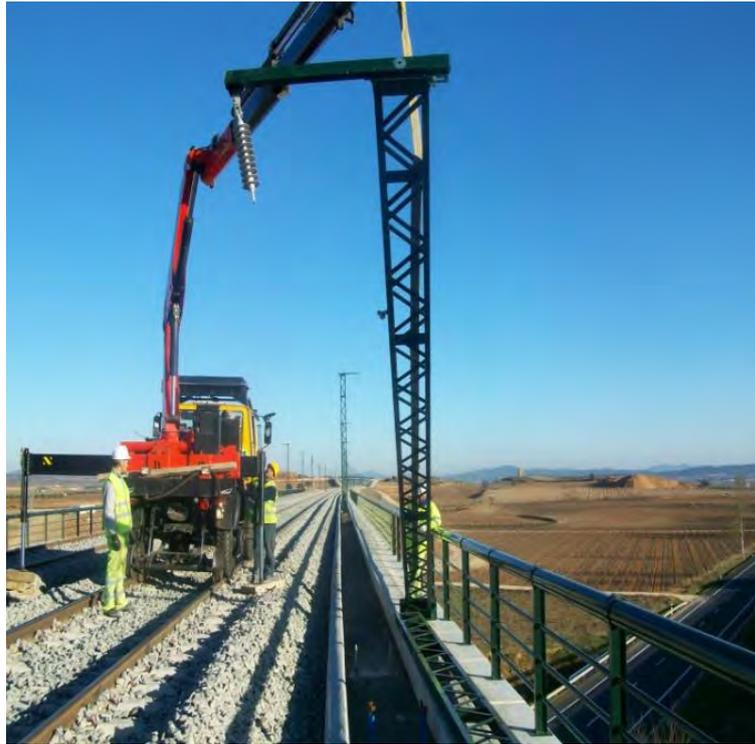
**Figure 5-81 Mast installation**
