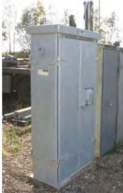
**Figure 5-72 Typical LOC (location case)**
