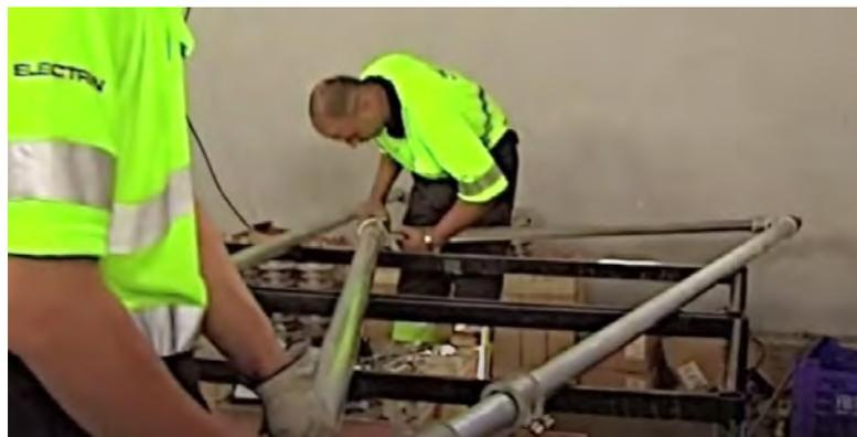
**Figure 5-84 Cantilever assembly**
