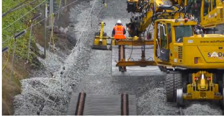
**Figure 5-19 Track panel installation**
