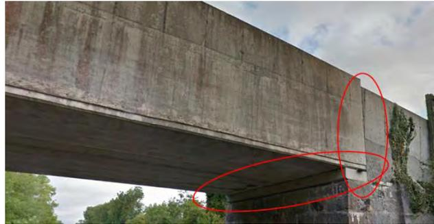
**Figure 5-390 Joints to be demolished at abutment**
