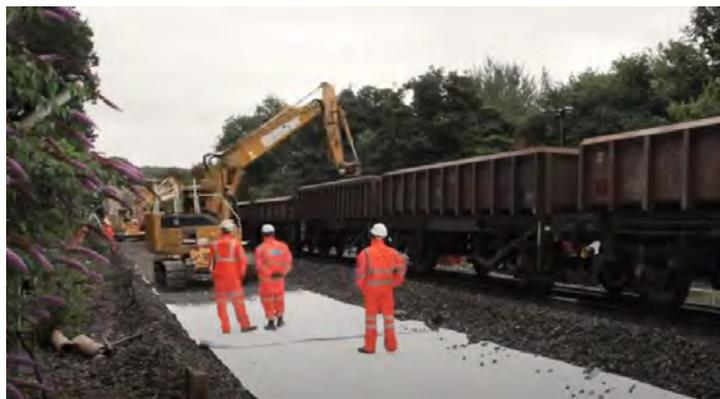
**Figure 5-17 Ballast laying**
