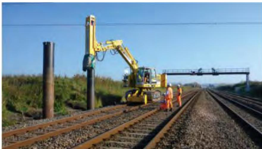
**Figure 5-79 Installation of steel piles**
