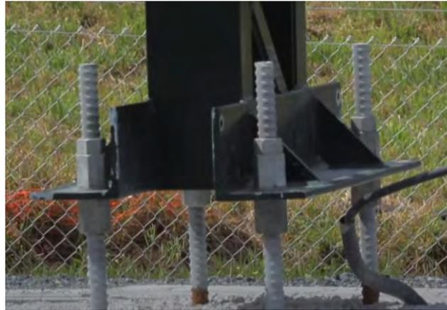
**Figure 5-83 Foundation anchor for masts**
