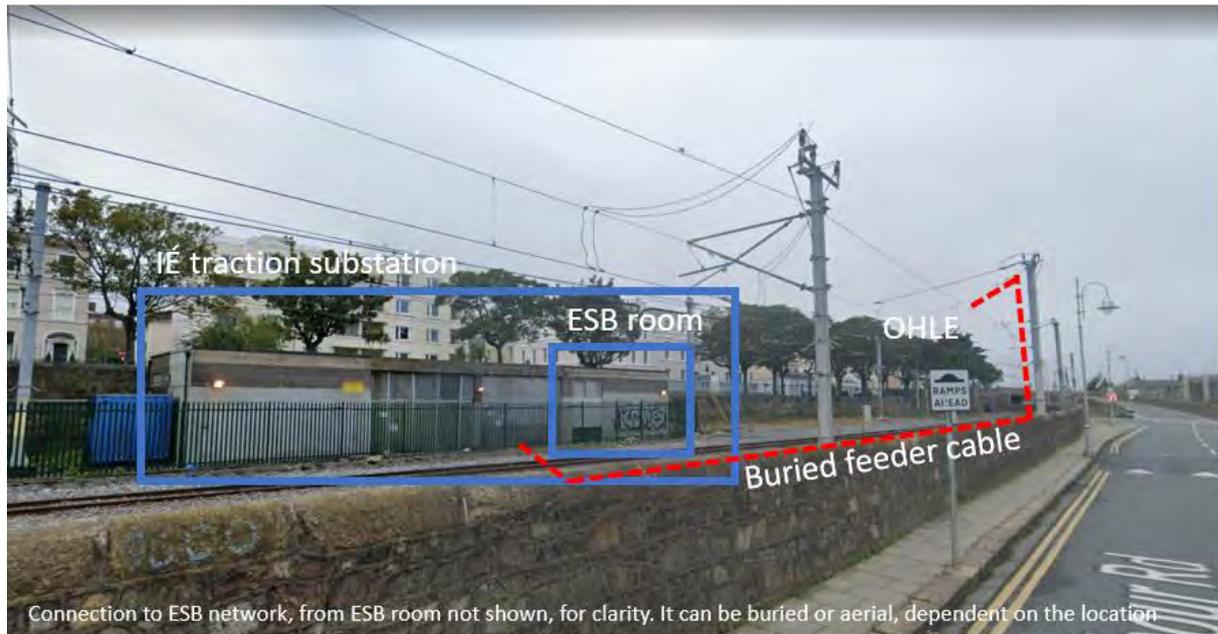
**Figure 5-62 Traction substation connections**
