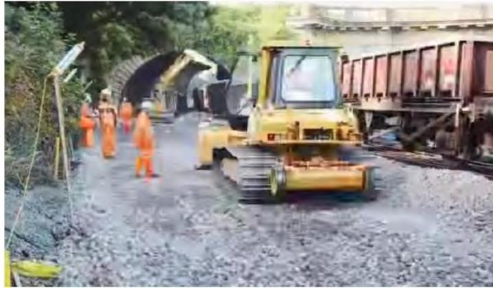
**Figure 5-25 Ballast laying and compaction**
