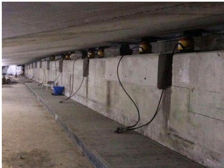
**Figure 5-56 Standard bridge jacking system**
