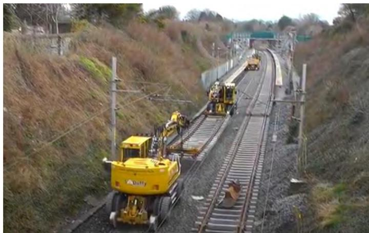
**Figure 5-14 Track panel removal**
