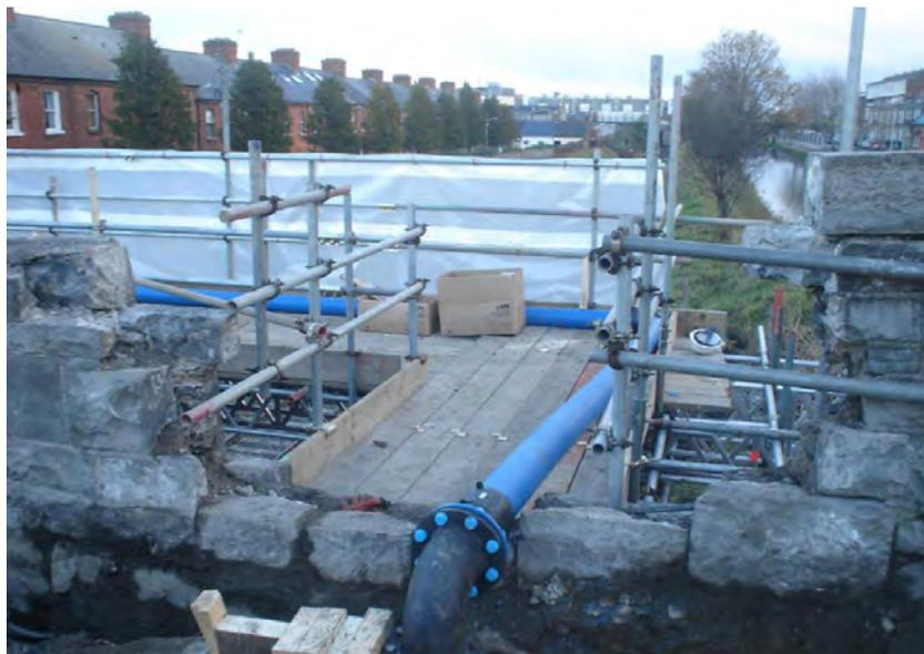
**Figure 5-7 Temporary diversion along scaffolding**
