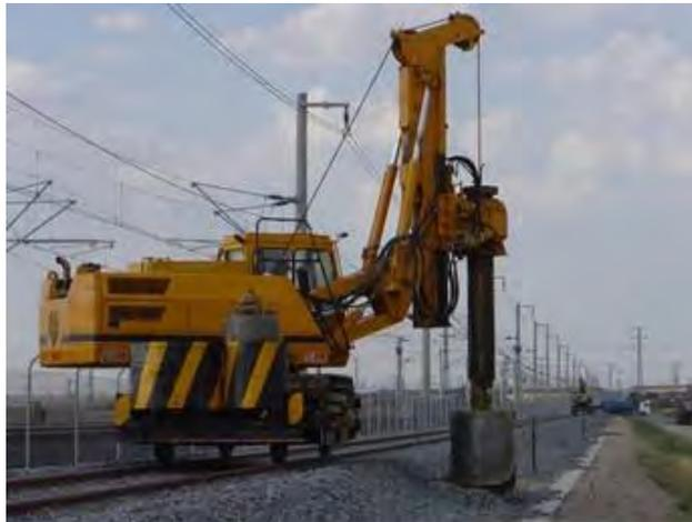
**Figure 5-77 Foundation drilling**
