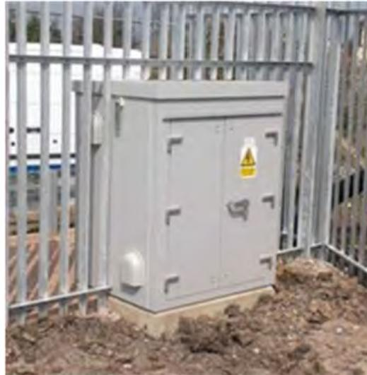
**Figure 5-67 Double sided DNO/distribution cubicle**
