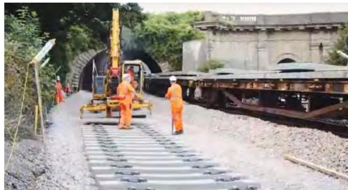
**Figure 5-26 Sleeper laying**
