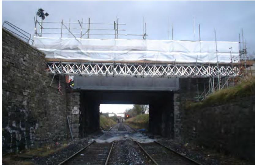
**Figure 5-6 Scaffolding for temporary diversion**
