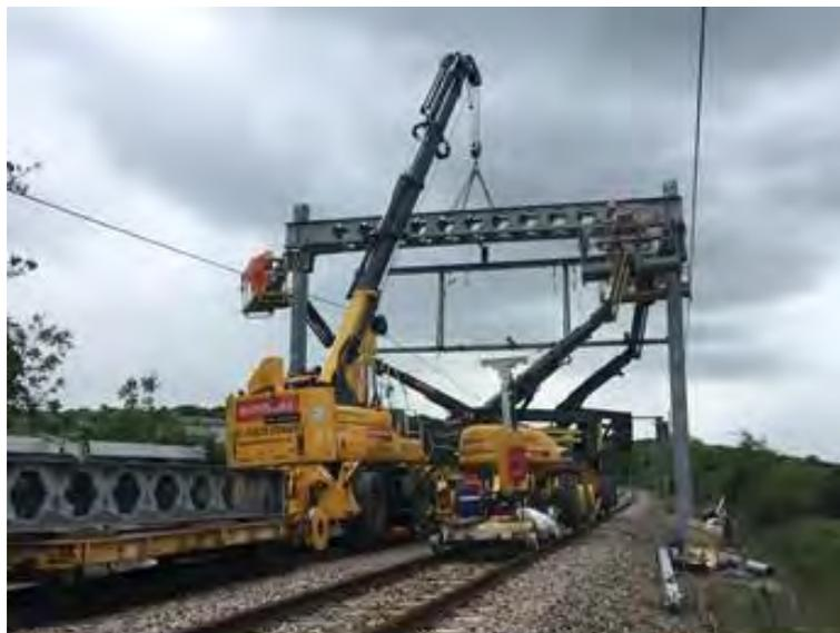
**Figure 5-82 Gantry installation**
