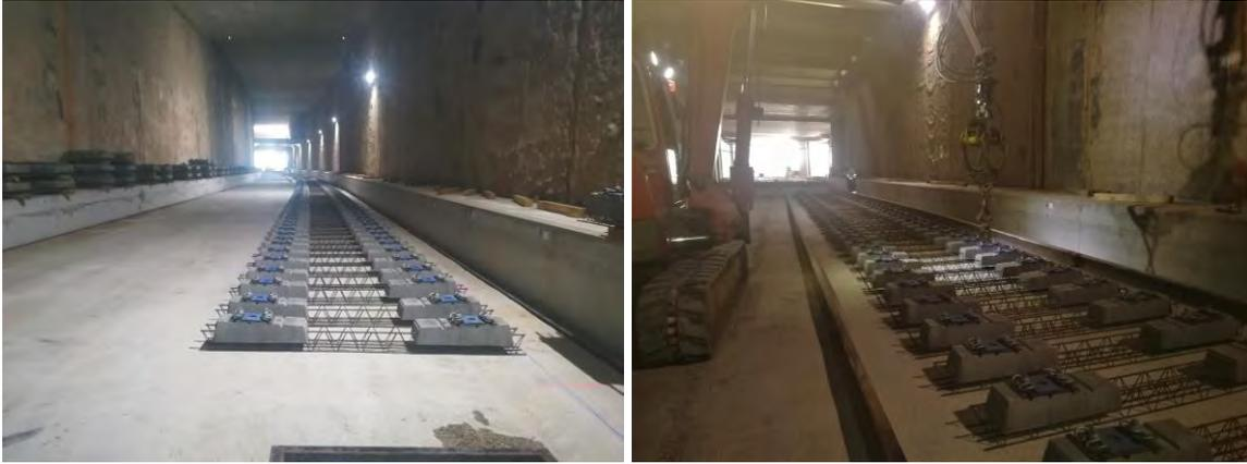
**Figure 5-29 Sleeper laying on top of structural slab**
