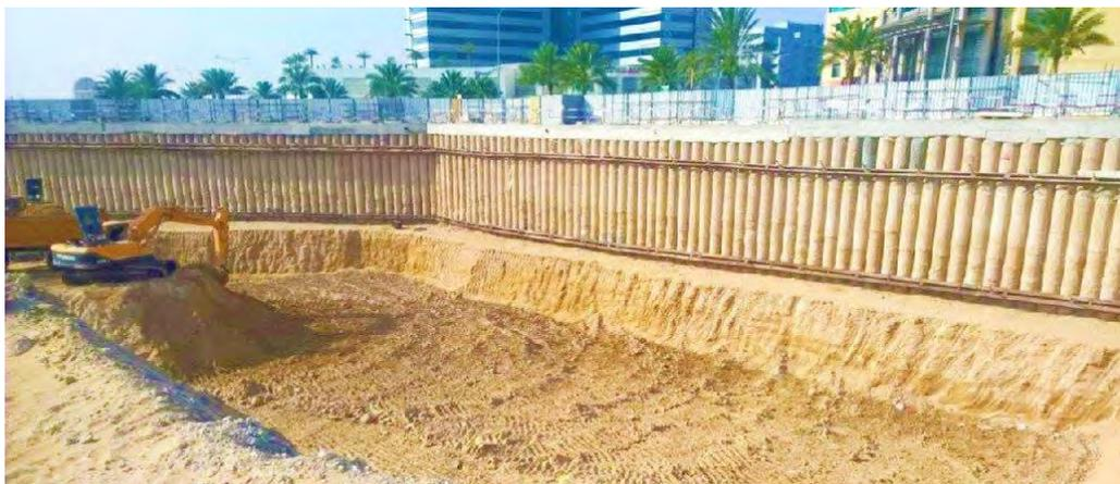
**Figure 5-202 Piled wall example**
