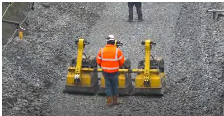
**Figure 5-18 Ballast compaction**
