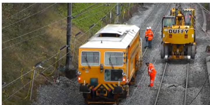
**Figure 5-22 Ballast tamping**
