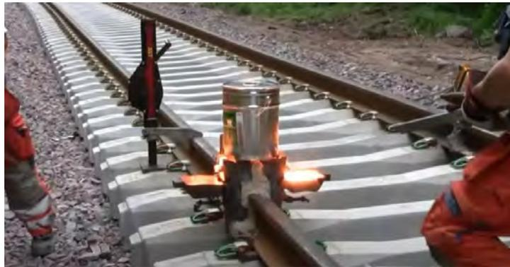
**Figure 5-23 Rail joint welding**
