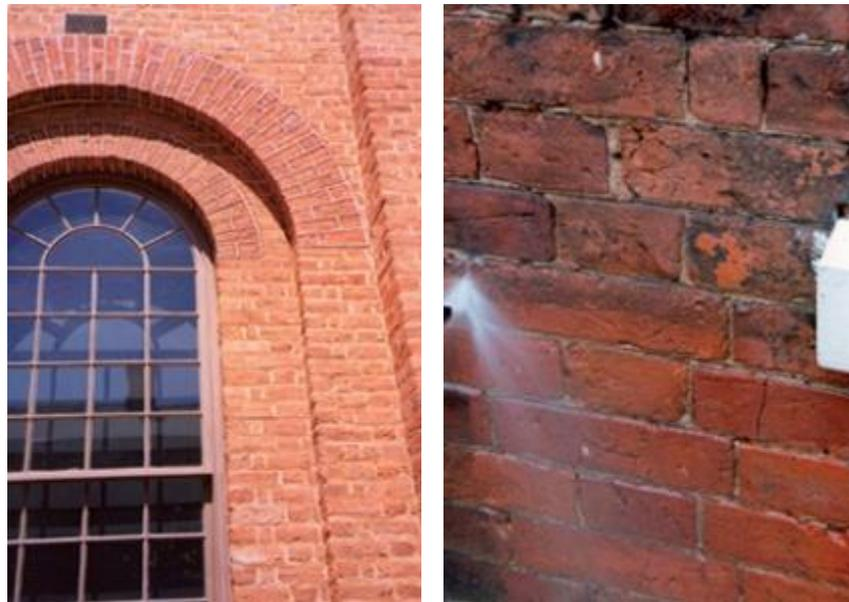
**Figure 32. Abrasive (left) and chemical (right) cleaning techniques**
