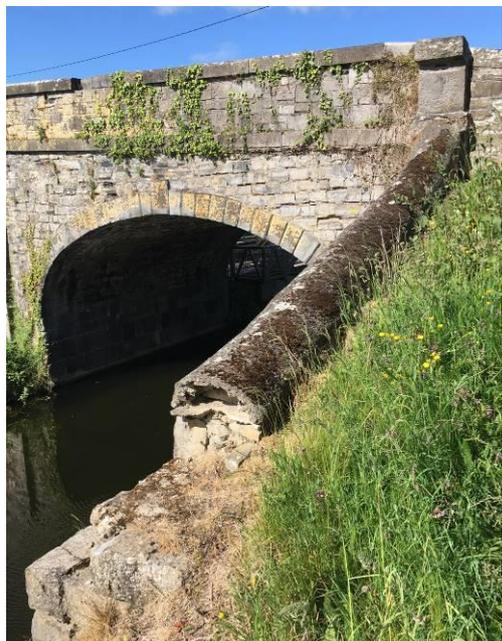
Figure 4 – North east wing wall with concrete flaunching.
