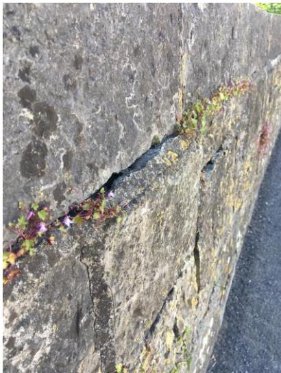
**Figure 24** – Mortar broken away from coping stone.
