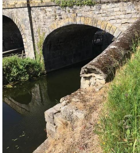
**Figure 23** – Top of pier lost, exposing end of modern concrete copings on north west wing.
