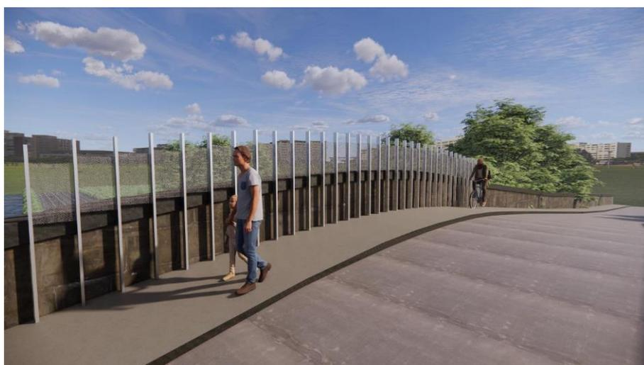
**Figure 32** – Render of design proposal to increase the parapet height to 1800mm with mesh about 1200mm.
