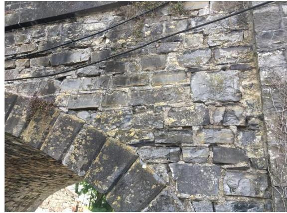
Figure 19 – Pointing loss on spandrel.
