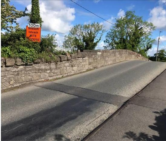
**Figure 12** – Road leading to the bridge from the south. The wall flanking the road is visible on the left. The crown over the railway arch and the bridge parapet are visible on the right.
