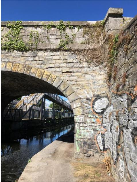
**Figure 9** – East facing spandrel of the canal arch showing squared limestone laid in slender courses.
