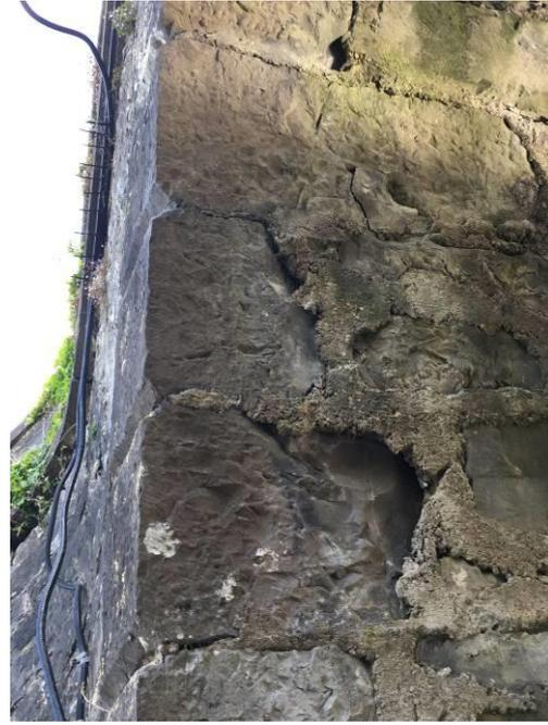
Figure 3 – Chamfer detail on arch voussoirs.
