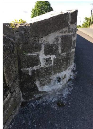
**Figure 26** – Recent repairs to north east corner.
