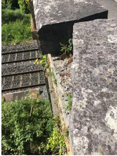
**Figure 27** – Lost section of coping stone over canal.
