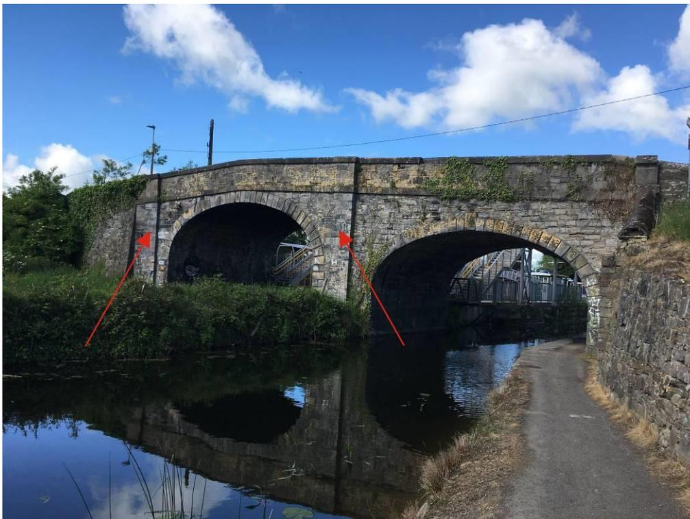
**Figure 30** - Existing bridge with piers highlighted. Existing bridge to be removed between piers.
