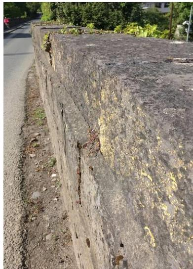
**Figure 25** – Coping does not extend to internal face of wall.
