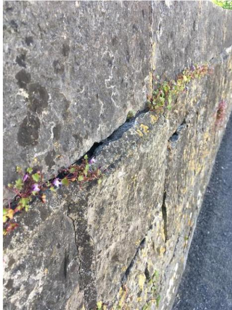
**Figure 33** – Stonework and pointing on parapet to be repaired.
