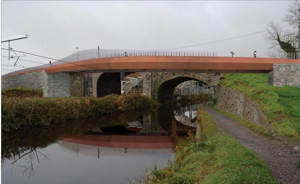
**Figure 34** – Proposed east elevation showing new pedestrian bridge and new concrete face over railway behind.
