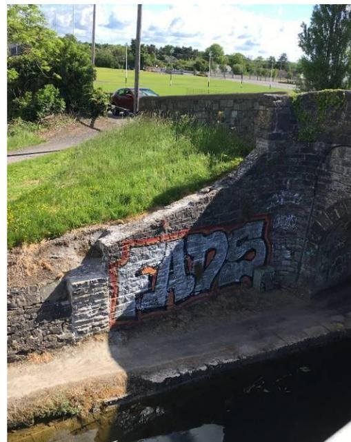
Figure 5 – North west wing wall with pier recently rebuilt. Note the wall is missing coping stones...
