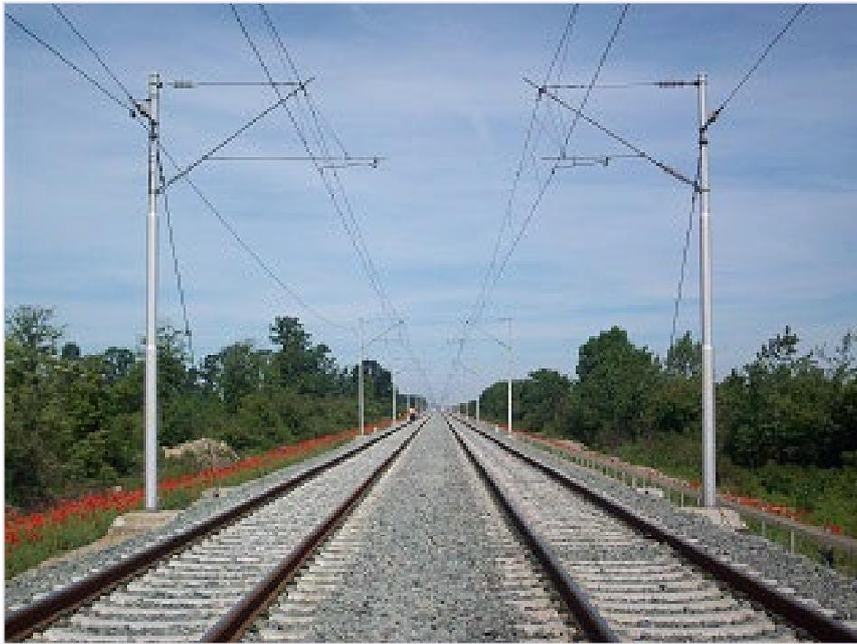
**Diagram 4.29: Example of Overhead Contact System**
