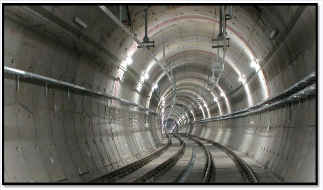
Diagram 4.28: Typical Example of an OCR in a Tunnel Section
