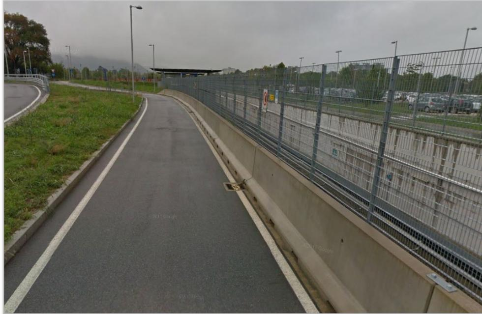
**Diagram 4.32: Example of Concrete Parapet and Fence**
