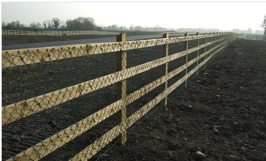
**Diagram 4.34: Example of a Timber Post and Wire Fence**
