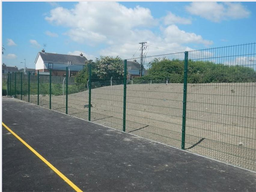
**Diagram 4.33: Example of 1.8m High Meshweld Fence**
