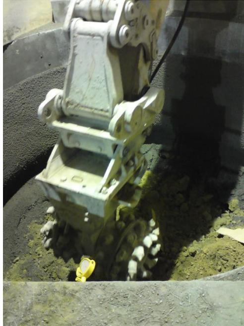
**Diagram 4.7: Example of Excavation of a Low Point Sump (A3, Hindhead Tunnel, Surrey)**
