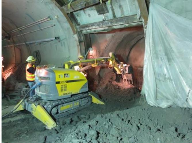
**Diagram 4.8: Break out of a Passage from a Main Tunnel**
