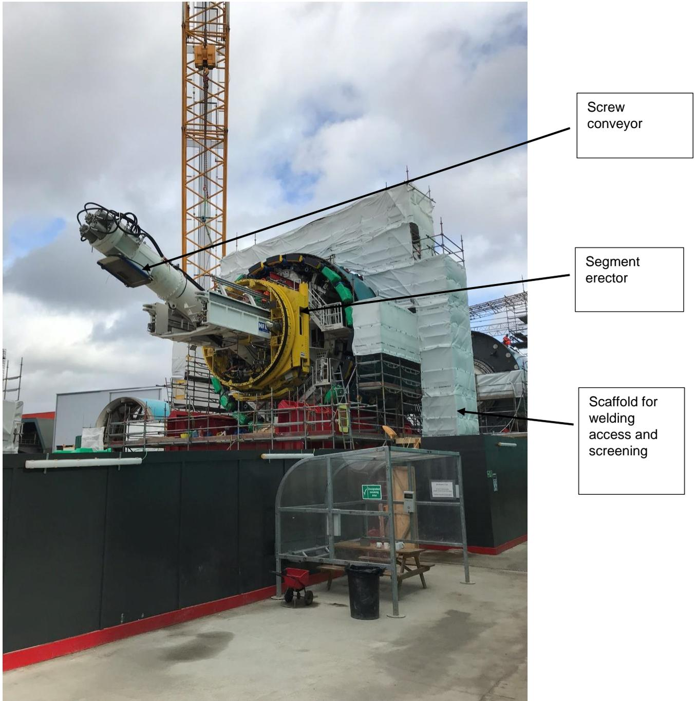
**Diagram 4.17: Segment erector and screw conveyor installed**
