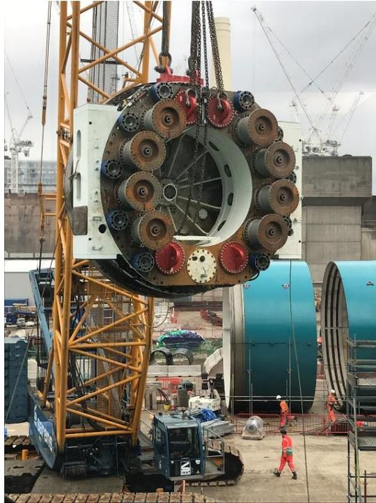
**Diagram 4.15: Drive module being lifted into place by a crawler crane**
