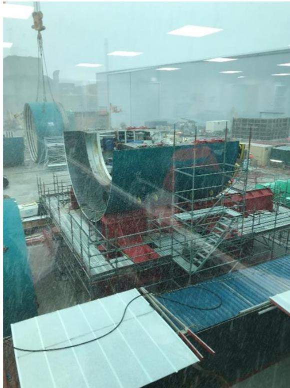
**Diagram 4.14: Front and middle shield bottom halves**
