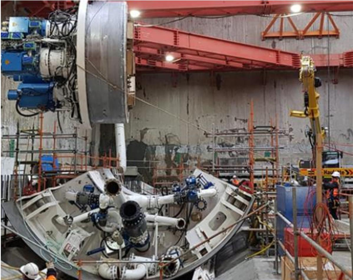
**Diagram 4.12: TBM Shield in Multiple Pieces**
