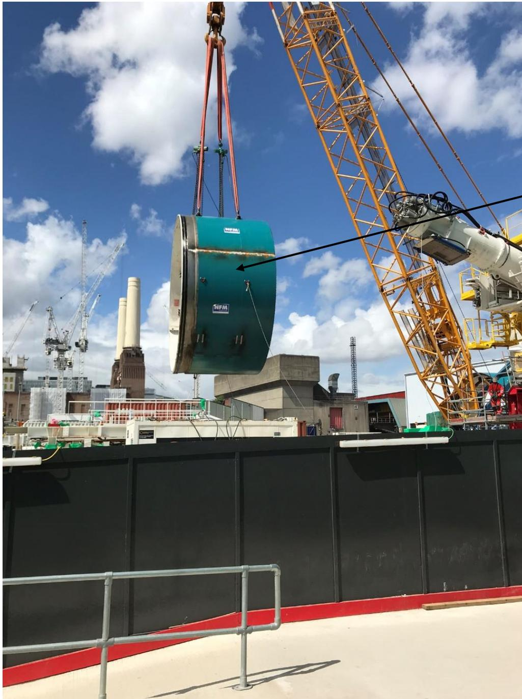
**Diagram 4.18: Tail shield being lifted into place. Note: it needs to turn 180 degrees before fitting to the middle shield**
