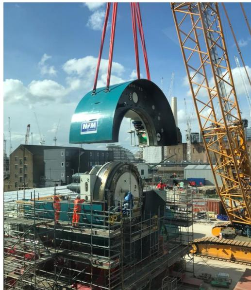
**Diagram 4.16: Front shield top half being lifted into place over the now-installed drive module**
