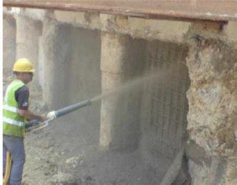
TamShot 10SS is used in sprayed concrete and annulus grouting applications which enables fast setting and/or where high early strength are required.
