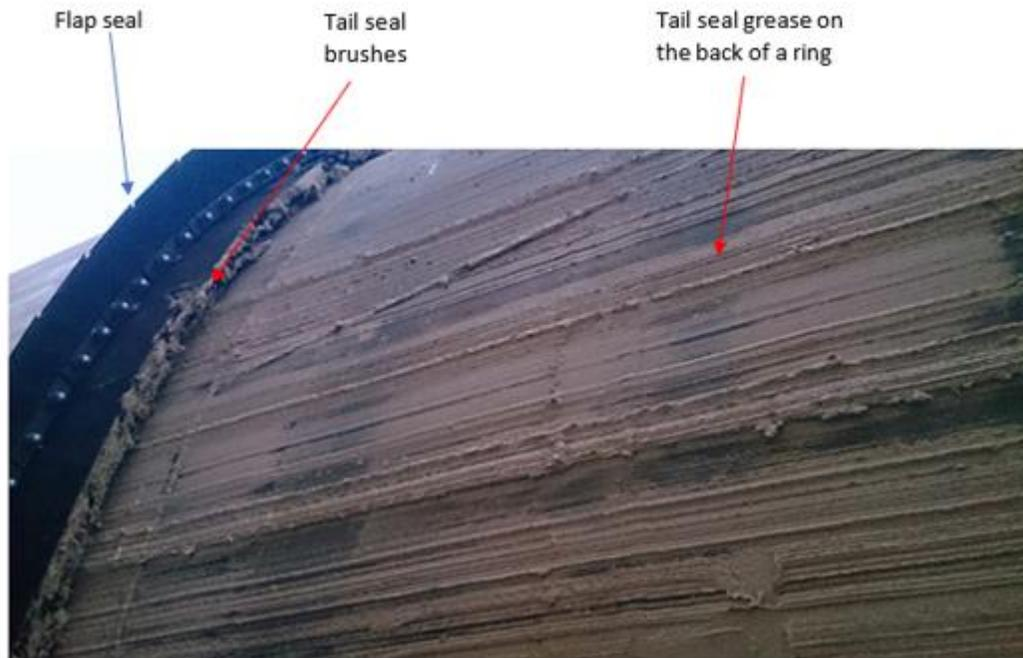
Diagram 2.9: Tail Seal Grease on the Outside of a Tunnel Ring
