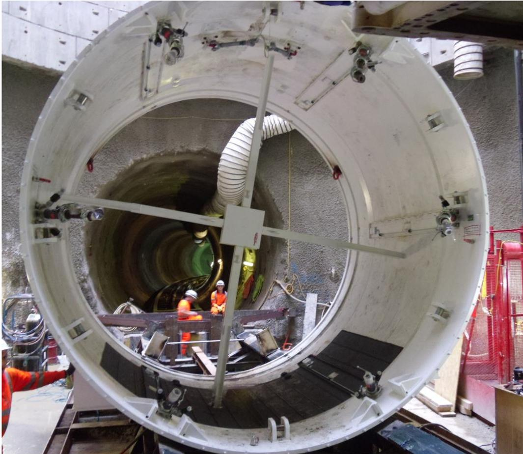
**Diagram 2.1: TBM Tail Can with Built-in Grout Tubes**
