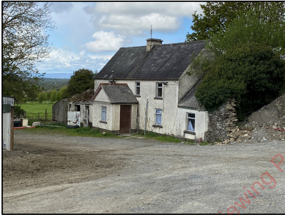
Plate 12.3 Structure 3 looking south-west.
