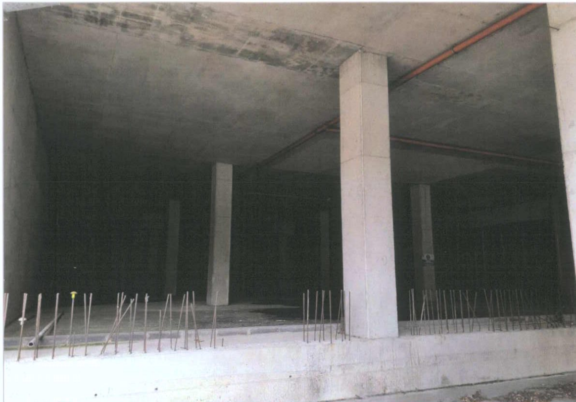
Figure 6.4.1.1 Much of the site is already built upon. September 2020.
