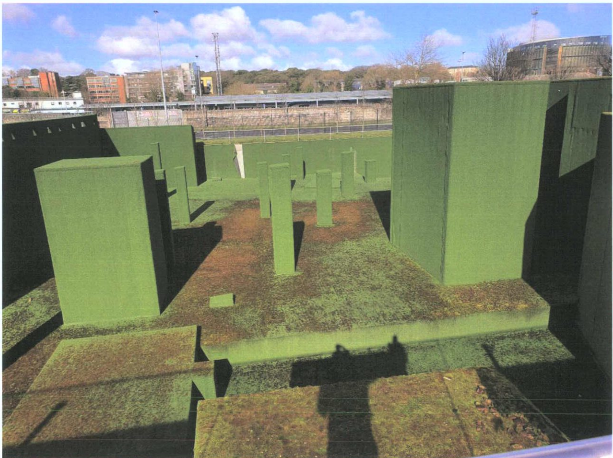
Figure 14.4.1.1 View from the subject site looking North
