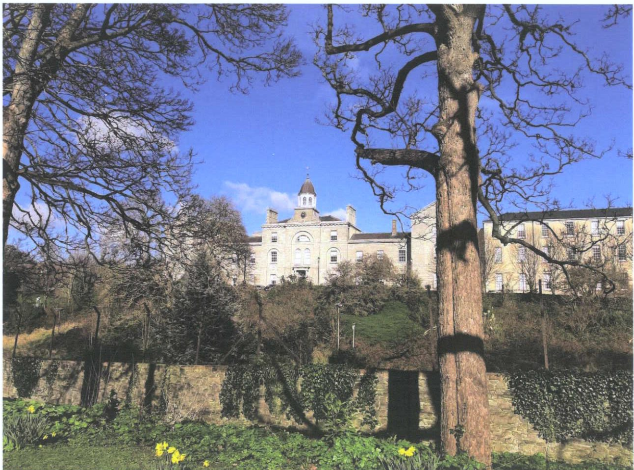
Figure 14.4.2.2.6 Former Military Hospital (Department of Defence)
