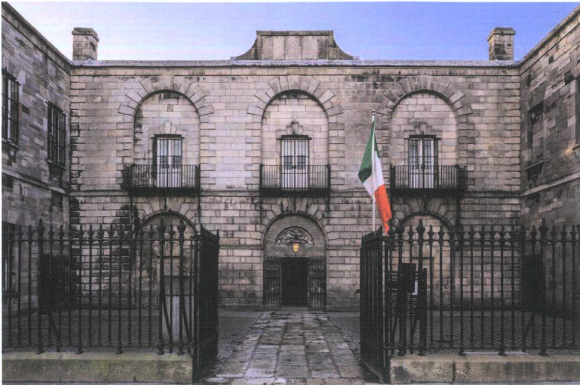
Figure 14.4.2.2.6 Former Gaol, Kilmainham
