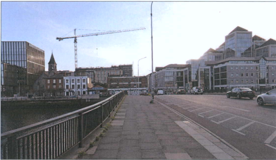
Photo 11.4 The existing site building facing Talbot Bridge and the Liffey, with the George's Quay office campus to the right, and two commercial premises, the Immaculate Heart of Mary Church and Grant Thornton.
