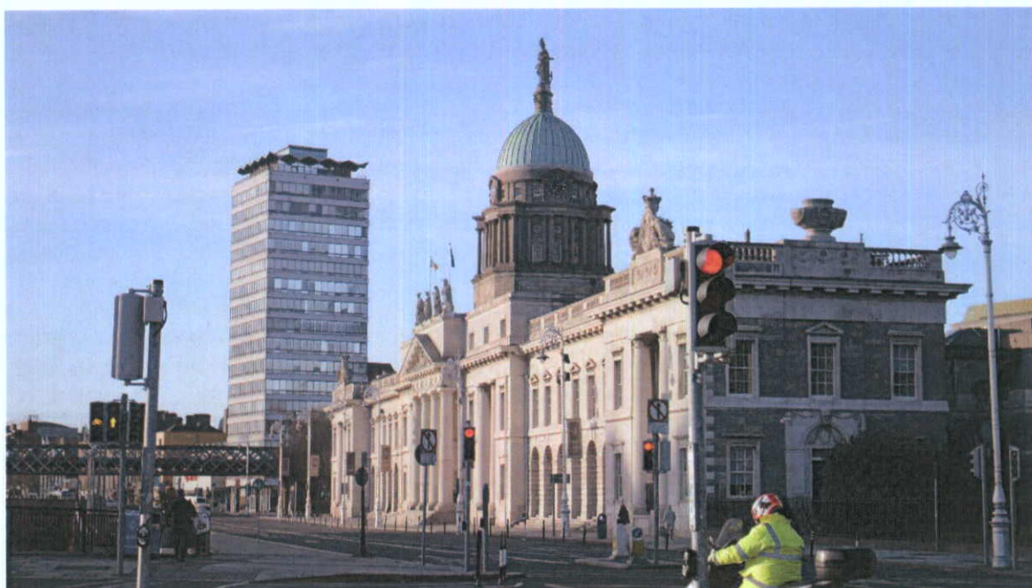
Photo 11.9 A view east along Custom House Quay showing Liberty Hall and the Loophouse bridge beside the protected structure. Although not tall, in footprint and overall massing the Custom House is a substantial building and it is surrounded by wide roads and the river. These factors allow it to accommodate other large buildings in its environs without being dominated.
