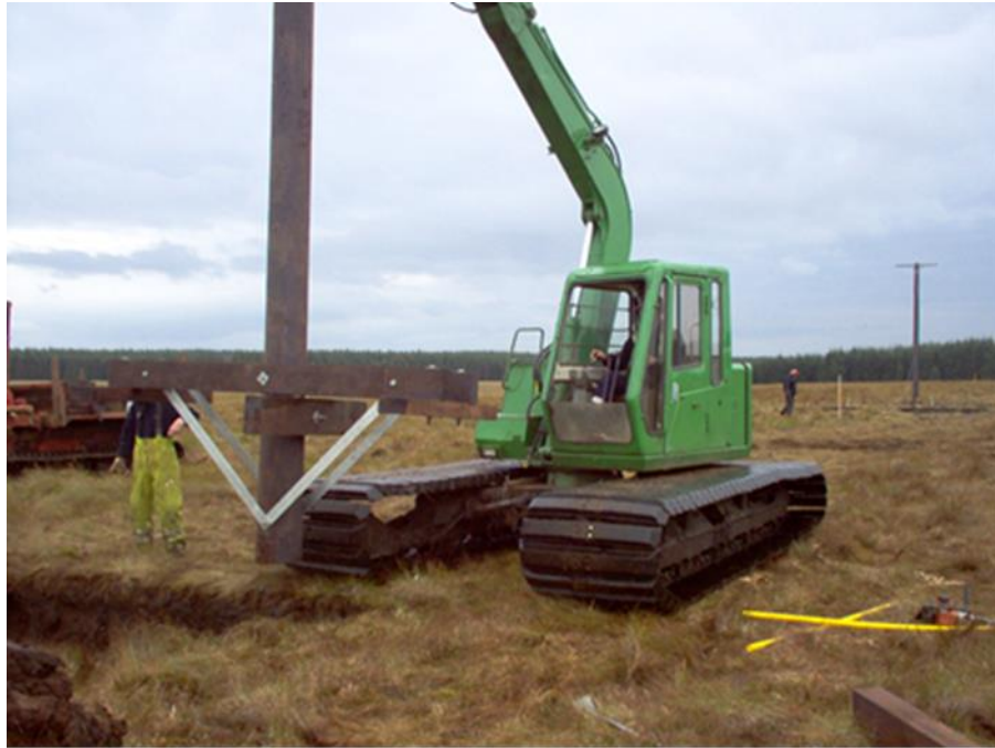
Plate 1 - Photograph of a Typical 20 kV Pole with Excavation
