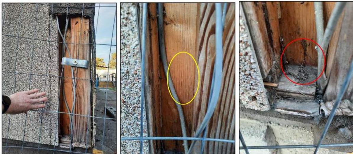
Figure 5-12 Images of the damage to pre-fab structure's south-western corner. Left-right: The damage, potential claw marks (Yellow) & insect remains at the base of the hole (Red).
