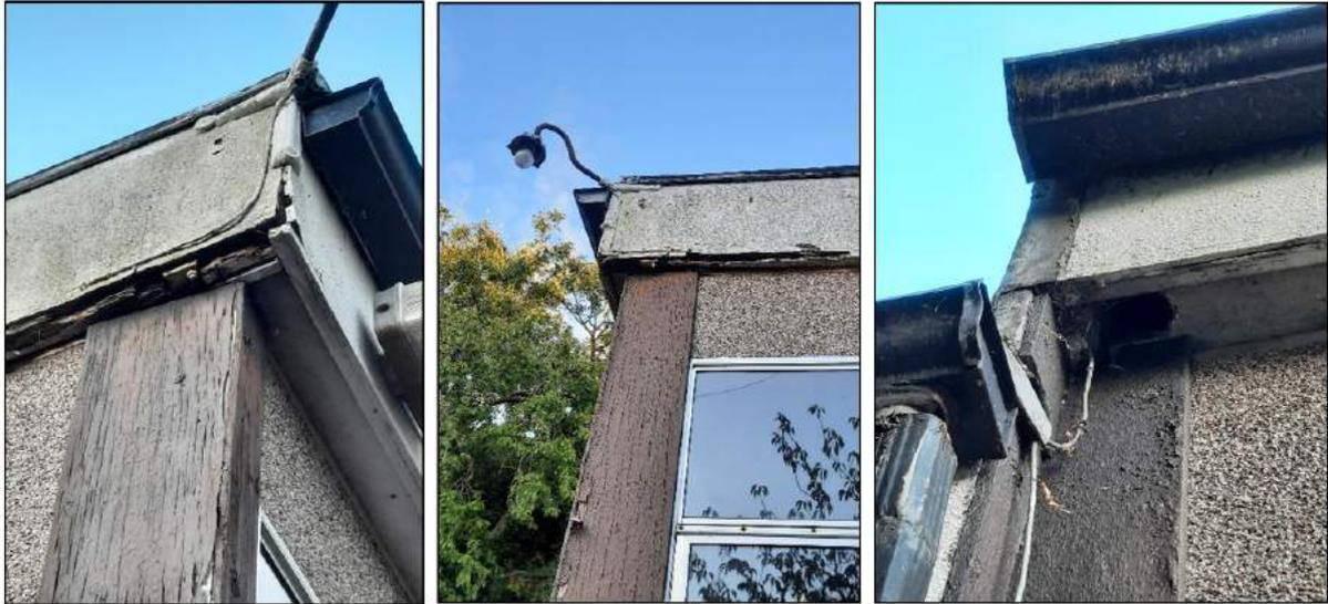
*Figure 5-9 Examples of PBR features observed at the prefab structure.*
