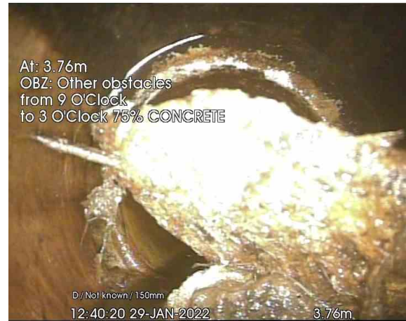
MH1 TO MH2_3-76m_124020.jpg, 00:00:27, 3.76 m Other obstacles from 9 o'clock to 3 o'clock, 75% cross-sectional area loss, CONCRETE
