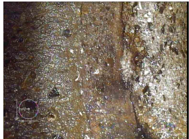
SMH3X_f949510e-b4f6-4394-8afe-2daf860bfc1d_20220408_101348_771.jpg, 00:02:23, 8.52 m Open joint, large
