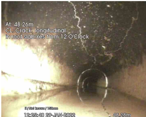
MH2 TO MH1_48-28m_122540.jpg, 00:04:41, 48.28 m Crack, longitudinal, in roof slab at 12 o'clock
