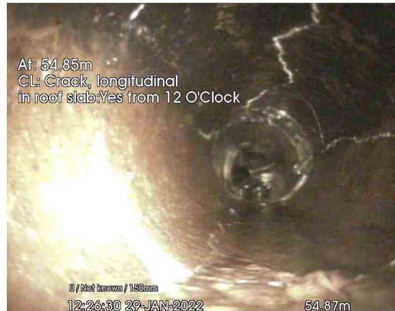
MH2 TO MH1_54-87m_122630.jpg, 00:05:14, 54.87 m Crack, longitudinal, in roof slab at 12 o'clock
