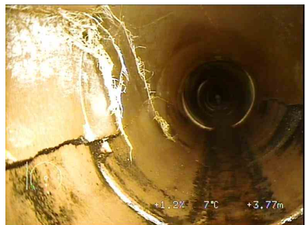
SMH4X_3e775cd6-07bf-448a-b8af-f02383adeace_20220408_124815_187.jpg, 00:00:56, 3.77 m Broken pipe at 9 o'clock
