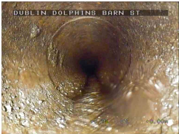
SMH2X_8c149130-048c-446d-86a1-1400bc3ca565_20220412_123830_327.jpg, 00:00:05, 0.00 m Attached deposits, other from 12 o'clock to 12 o'clock, 5% cross-sectional area loss, finish, SILT
