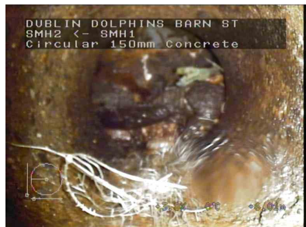
SMH2X_d3a5553c-1358-44da-8de2-f74cbf6eea60_20220408_100312_296.jpg, 00:02:22, 6.01 m Junction at 9 o'clock, 100mm dia
