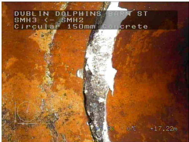
SMH3X_2856e269-1400-4a1e-880a-86ee3f0c09ed_20220408_102207_967.jpg, 00:06:36, 17.22 m Fracture, circumferential at joint from 10 o'clock to 12 o'clock
