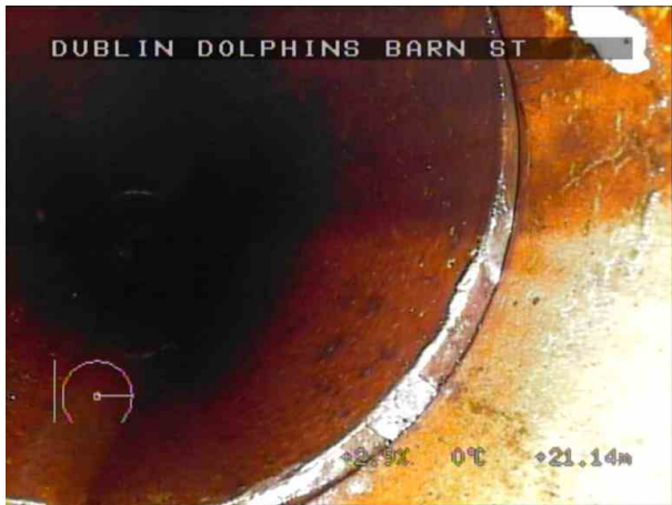
SMH3X_b2ac8f39-db7c-4314-b07c-01876c25bebb_20220408_102842_873.jpg, 00:08:54, 21.14 m Joint displaced, large
