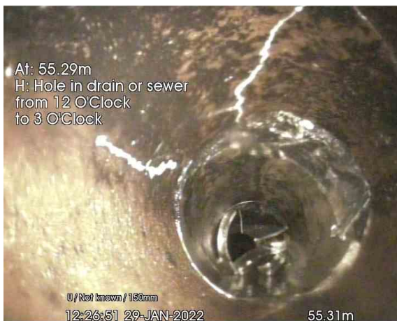
MH2 TO MH1_55-31m_122651.jpg, 00:05:26, 55.31 m Hole in drain or sewer from 12 o'clock to 3 o'clock
