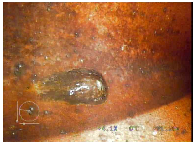
SMH3X_d48bc823-7a6c-4735-a61d-b64428dd3433_20220408_102923_372.jpg, 00:09:18, 21.20 m Deformed sewer or drain, 5%
