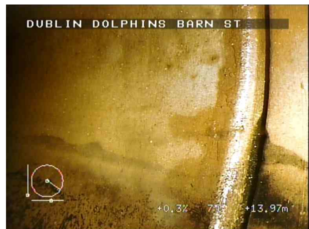
SMH4X_f82a13ab-69c4-45fd-8f68-8b0b8f6aada8_20220408_125015_918.jpg, 00:02:34, 13.97 m Open joint, medium
