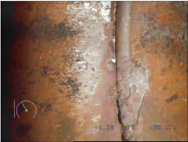
SMH3X_2d4f37a4-ef05-4947-9a4c-4fce43f26fed_20220408_103232_340.jpg, 00:11:25, 28.37 m Deformed sewer or drain, 10%
