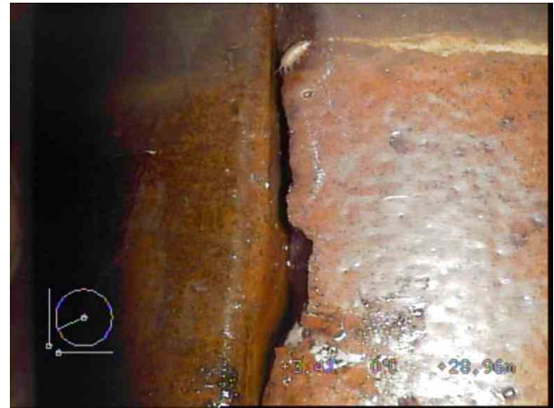
SMH3X_c4e3b749-1326-407f-856d-6befd816f5e4_20220408_103324_828.jpg, 00:12:01, 28.96 m Open joint, large
