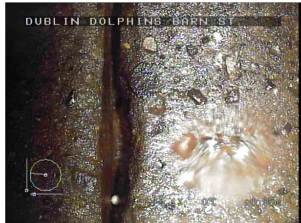
SMH2X_0889b6b3-45e6-4b41-bbfa-a42acf304ac4_20220408_100034_943.jpg, 00:00:27, 0.85 m Open joint, medium
