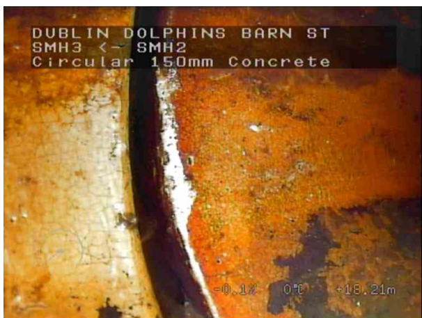
SMH3X_4560511f-a8a0-4761-b103-2ad8f21897b7_20220408_102426_372.jpg, 00:07:51, 18.21 m Open joint, medium
