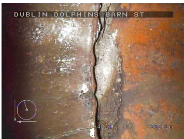
SMH3X_e097369b-9d07-4f80-b9f6-642262c70cb6_20220408_103357_091.jpg, 00:12:25, 29.61 m Open joint, large
