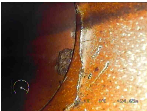
SMH3X_0ebb6a48-de9d-4969-8cc3-2cbcd6f102d8_20220408_103035_844.jpg, 00:10:19, 24.65 m Crack, circumferential from 3 o'clock to 4 o'clock
