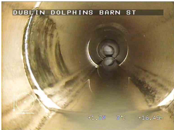
SMH4X_640e99a1-0852-4f0b-bc90-f30d2a366878_20220408_125041_365.jpg, 00:02:54, 16.45 m Joint displaced, large
