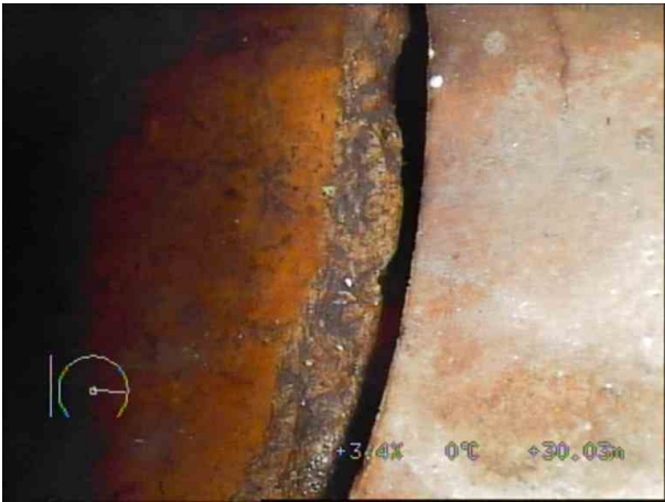
SMH3X_0aac7fce-5a23-446e-884d-486e70784976_20220408_103502_848.jpg, 00:13:00, 30.03 m Open joint, large
