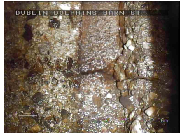
SMH3X_191414e8-b719-45b2-aca3-856292a3ef3b_20220408_101720_789.jpg, 00:04:57, 15.06 m Open joint, large, CRANCK ON JOINT
