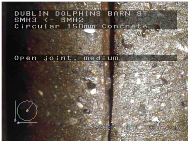
SMH3X_ee8eff8b-ef12-4309-8494-48da32b7e79d_20220408_101528_559.jpg, 00:03:34, 10.49 m Open joint, medium
