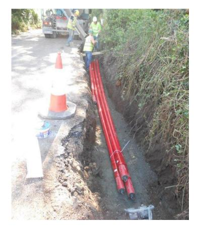
Figure 3-10: Cable Duct Laying in Trefoil Configuration
