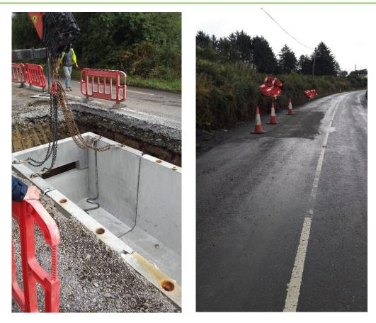
Plate 3-6: Typical Installation and Temporary Reinstatement of Joint Bay
