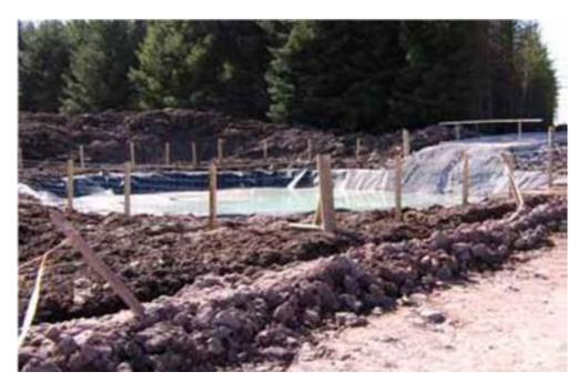
Figure 4-8: Lined Settlement Lagoon for Concrete Washout Facility
