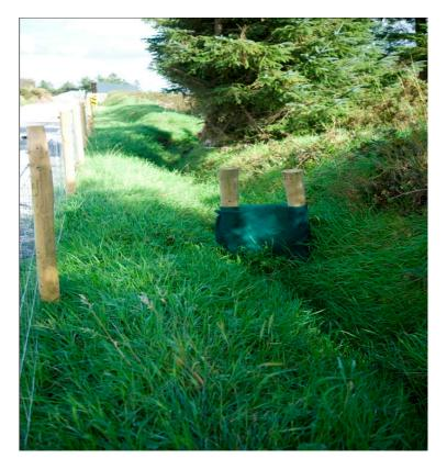
Figure 4-4: Silt Trap across Grassed Swale
