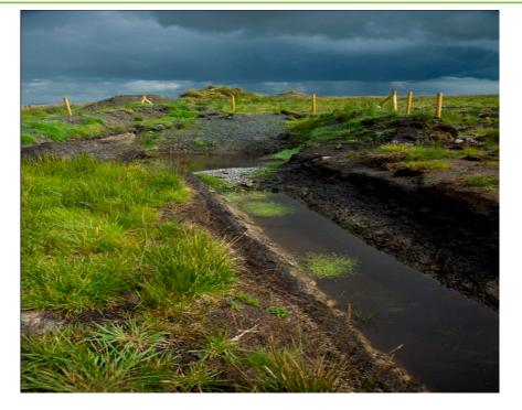
Figure 4-2: Swale draining to Settlement pond
