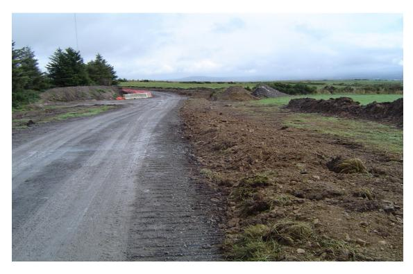
Figure 4-7:Backfill over Cable Trench
