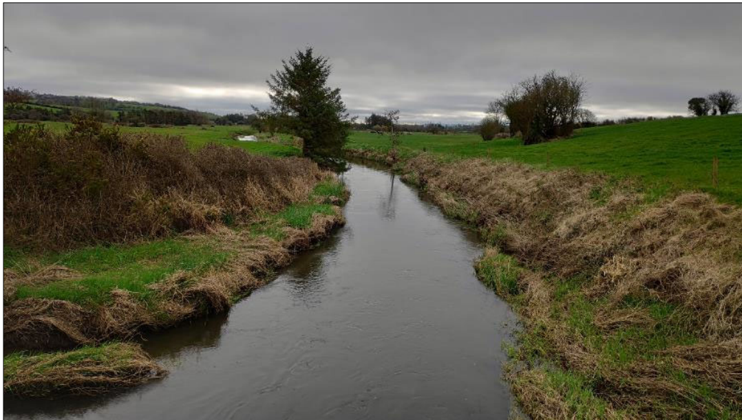
Plate 3.6 Representative image of the Awbeg River at Scart Bridge (site A3), demonstrating historically straightened and deepened channel
