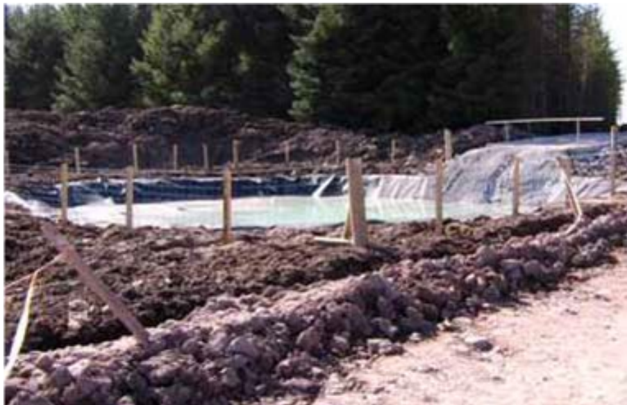
Figure 3-9: Lined Settlement Pond for Concrete Washout Facility
