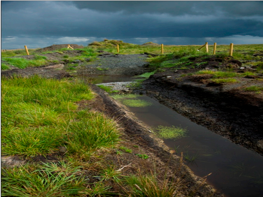
Figure 3-3: Swale draining to Settlement pond
