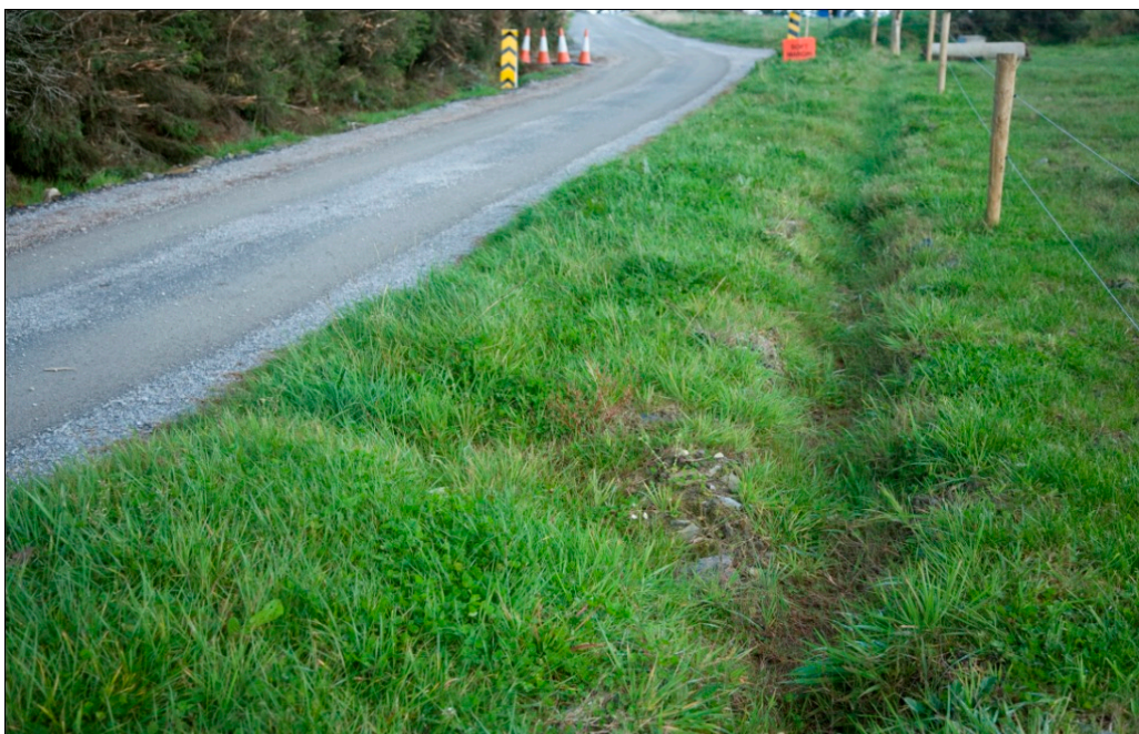
Figure 3-2: Grassed swale along access track
