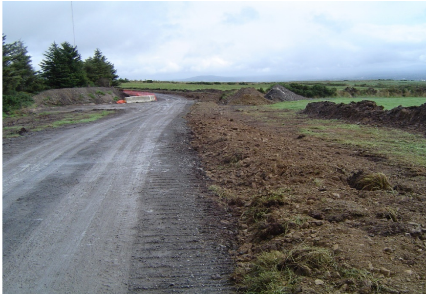
Figure 3-8: Backfill over cable trench
