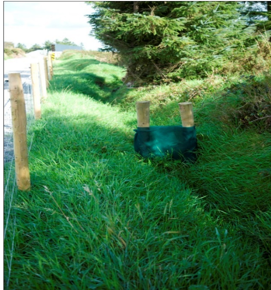
Figure 3-5: Silt trap across grassed swale
