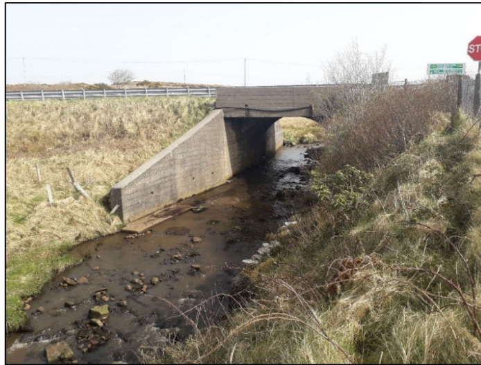
Figure 10 - Bridge 2 within the N59
