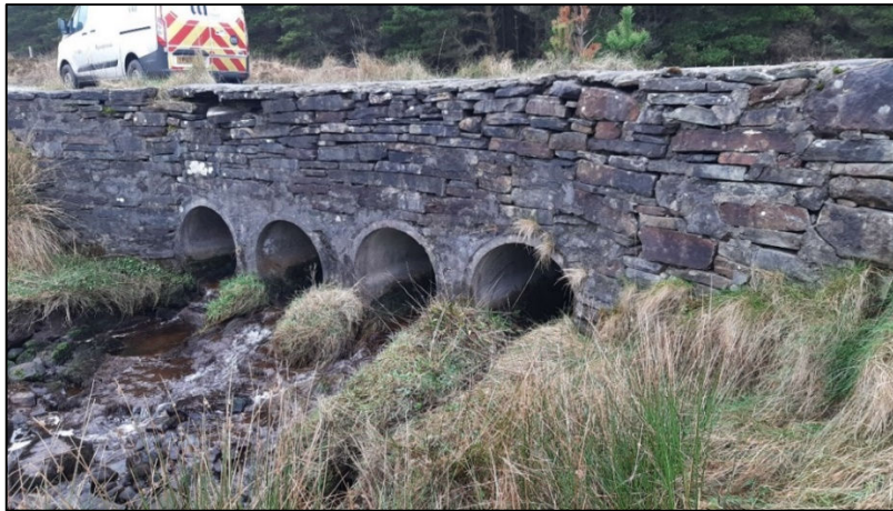
Figure 12 - Bridge 3 within the forestry access roadway
