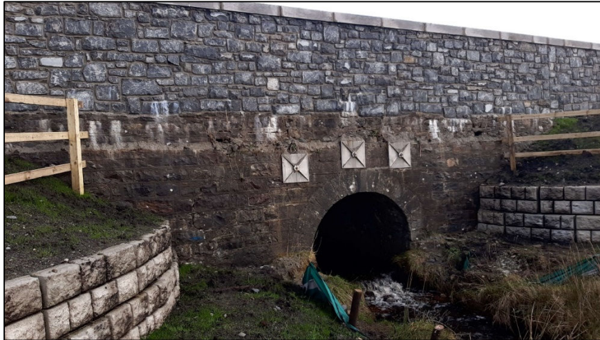
Figure 8 - Bridge 1 within the N59
