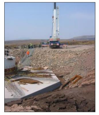
Plate 6.1: Turbine foundation under construction with adjoining crane pad<sup>5</sup>
