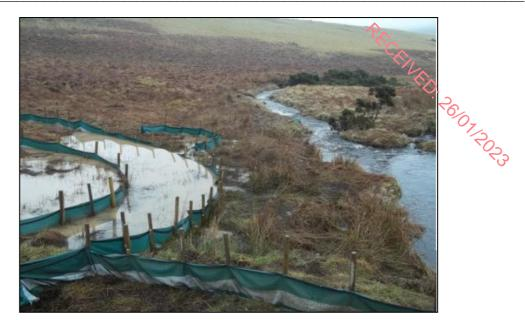
Plate 1: Photograph of Silt Fencing
