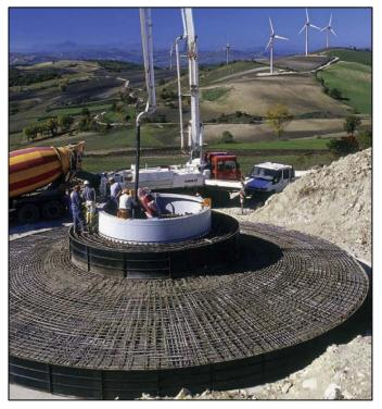
Plate 6.2: Wind turbine foundation<sup>6</sup>
