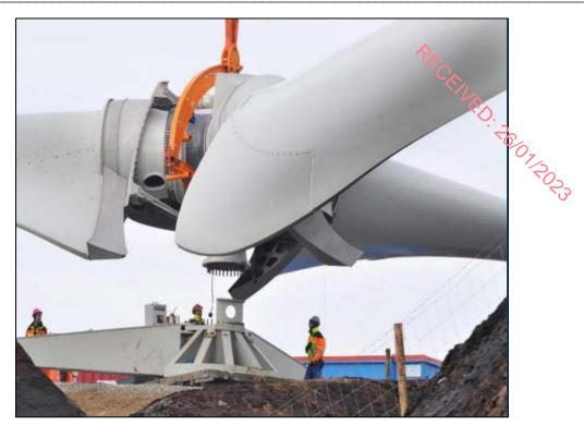
Plate 6.4: Assembly of wind turbine blades <sup>2</sup>
