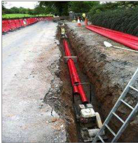
Figure 5 – Typical 38kV Underground Duct Installation
