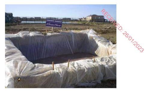
Plate 2.3: Typical Temporary Concrete Washout Area
