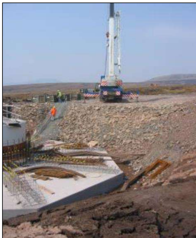
Plate 6.1: Turbine foundation under construction with adjoining crane pad 5
