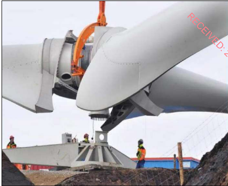
Plate 6.4: Assembly of wind turbine blades 2
