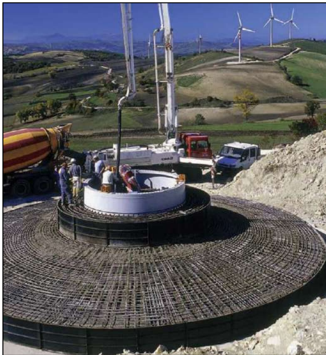
Plate 6.2: Wind turbine foundation 6
