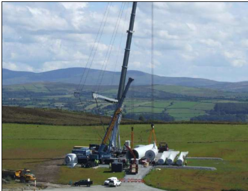
Plate 6.3: Wind Turbine Erection 2
