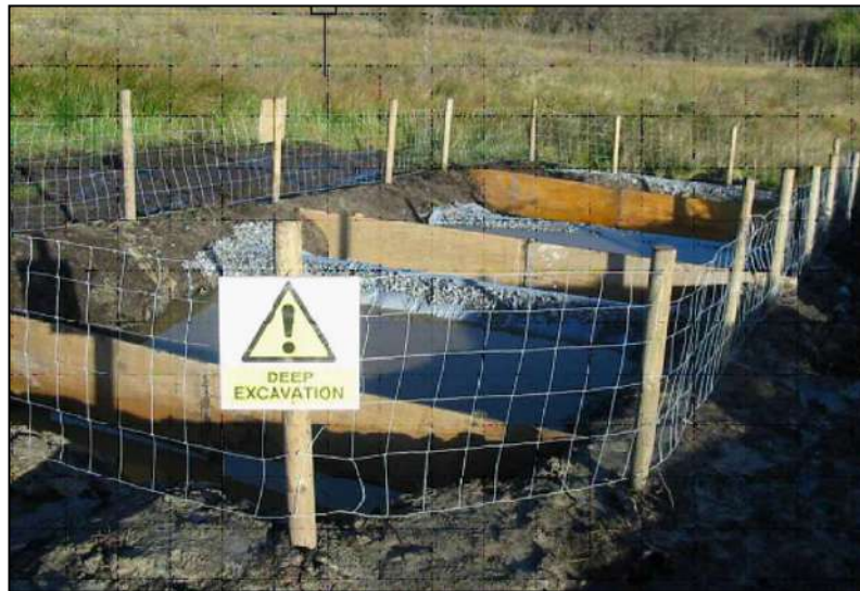
Plate 2: Completed Settlement Pond System
