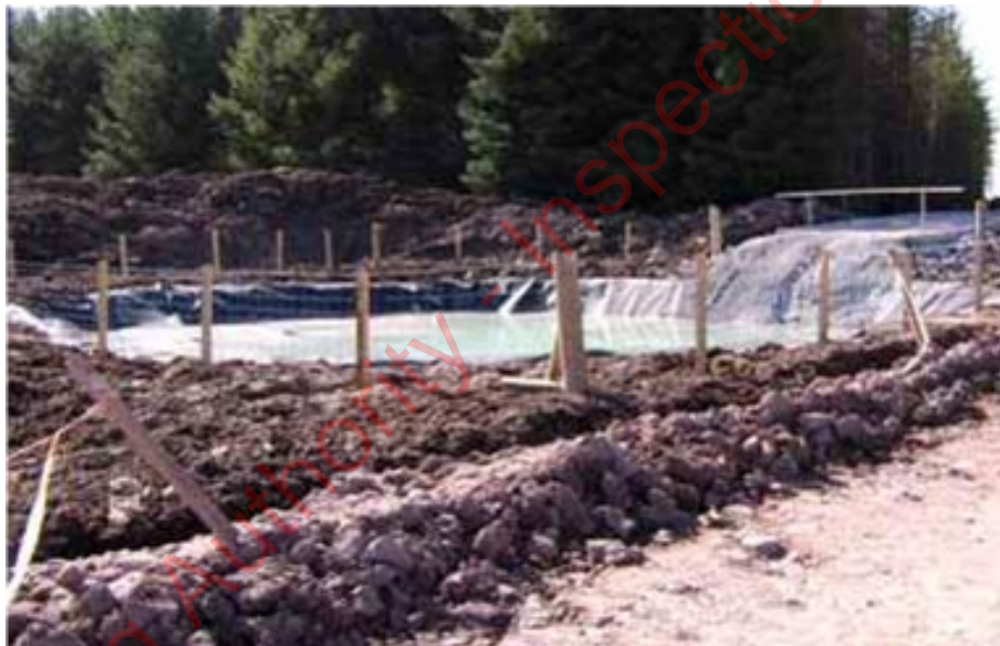
Figure 3-9: Lined Settlement Lagoon for Concrete Washout Facility
