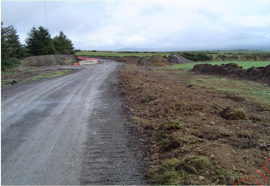
Figure 3-8: Backfill over cable trench
