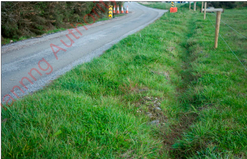
Figure 3-2: Grassed swale along access track
