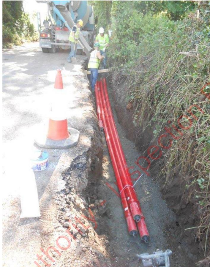
Plate 3-1: Cable Duct Laying in Trefoil Configuration
