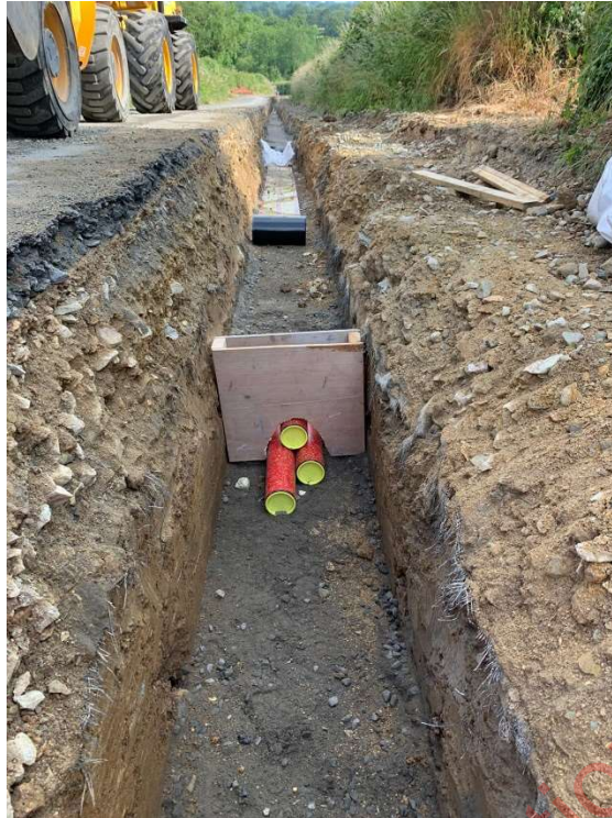
Figure 5 - Typical 38kV Underground Duct Installation
