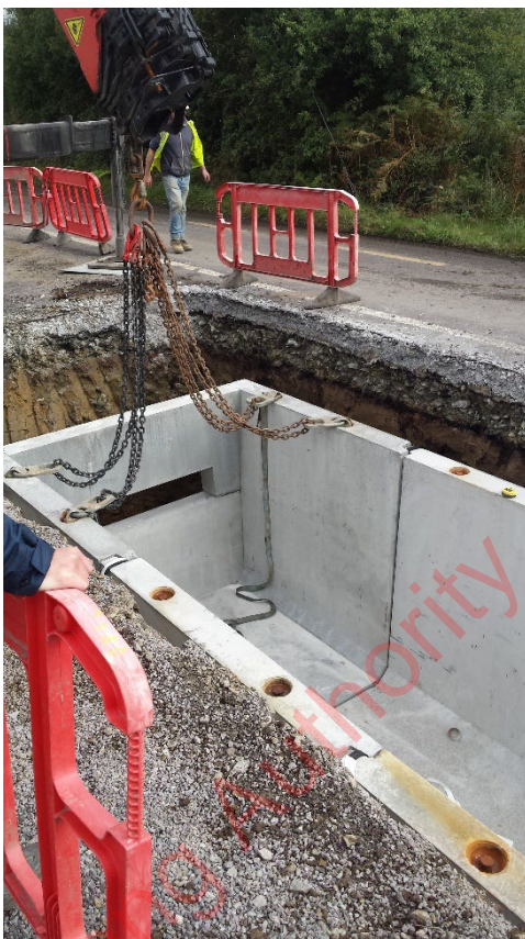
Figure 3-8: Typical Installation and Temporary Reinstatement of Joint Bay
