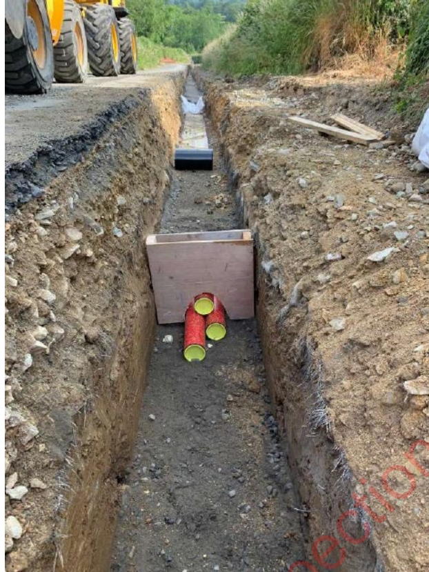
Figure 3-7: Typical 38kV Underground Duct Installation
