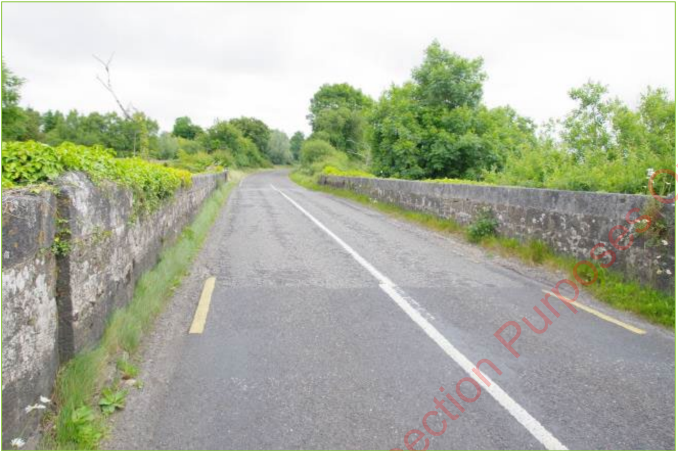
Plate 14-15: View of Aharinaghbeg road bridge along grid connection
