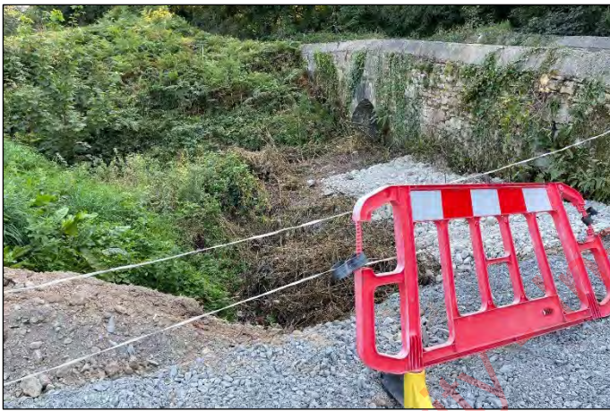
Plate 8 Alternative view of Survey Site A3 showing extensive works taking place.
