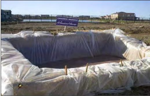
Plate 4-1 Concrete washout area
