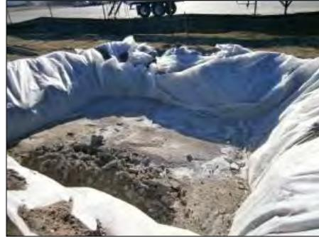
Plate 4-2 Concrete washout area
