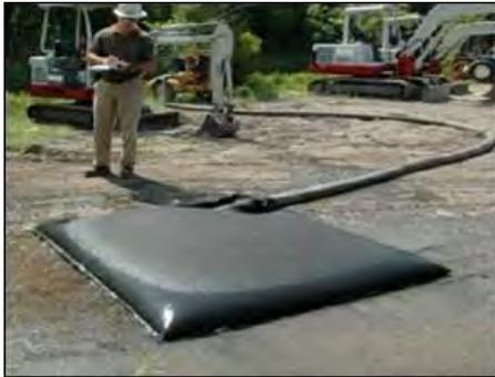
Plate 4-3 Silt Bag with water being pumped through
