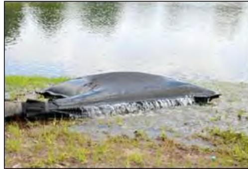
Plate 4-4 Silt bag under inspection
